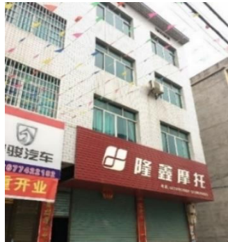
Figure 1: View of the case building in Hunan, China
