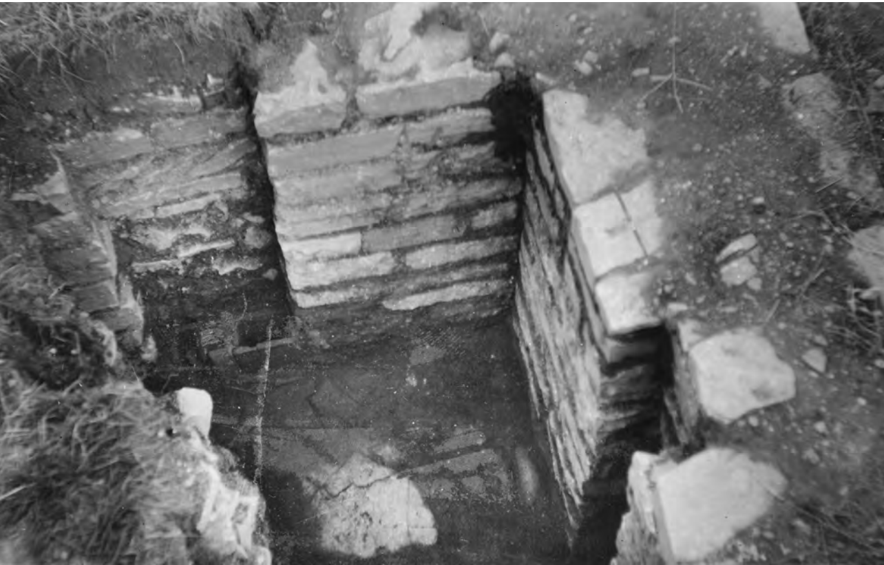
Fig 3.22 Looking south-west to the south-west inside corner of Room 19, with recesses for box-flue tiles visible on both walls. One such tile appears to remain in situ (HEA RAD01/22/12/009)
