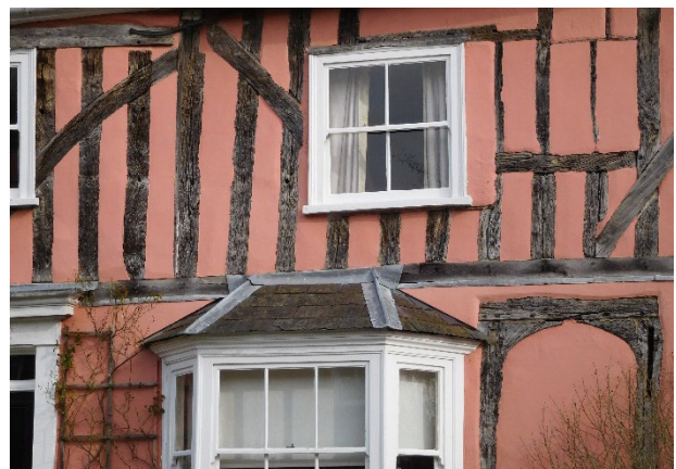
Figure 1. C15 timber-framed building, "Cordwinders", High St, Lavenham, Suffolk (Author, 2017)
