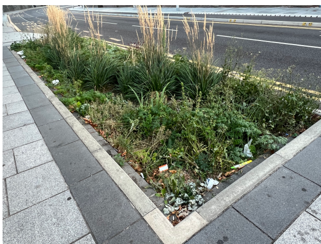
Figure A.4 Station Terrace biofilters.
