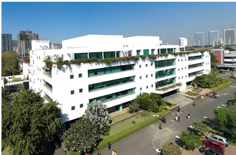
Figure 3. Godrej Plant 13 Annexe, Mumbai.
