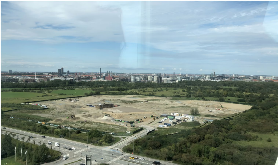
FIGURE 1 The Fælledby construction site, with the wall around it clearly visible (photo by the author, 13 September 2023).
