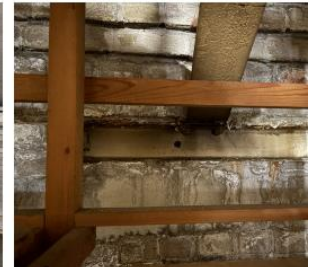
292. Health wing Attic wall
