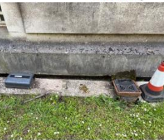
79. North corner facade dropped ground level
