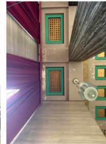
164. G04 Ceiling at North corner.
