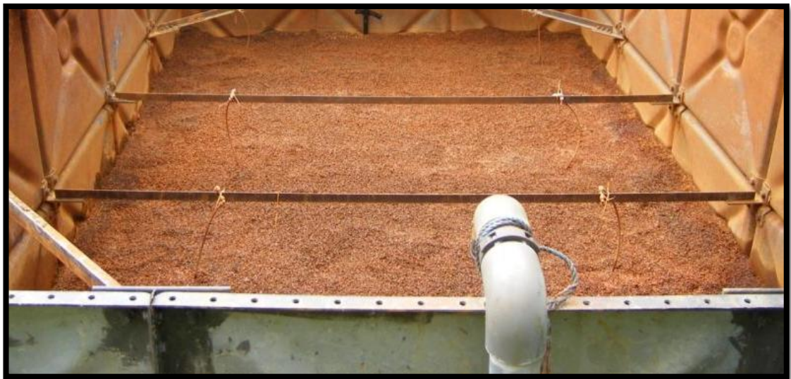
Figure 4-14 The VFR after cleaning, 7cm deep layer of sludge has been removed.
