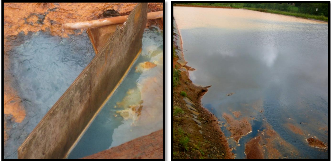
Figure 3-2 Calcium carbonate dosing at Blenkinsopp showing blue \text{FeCO}_3
