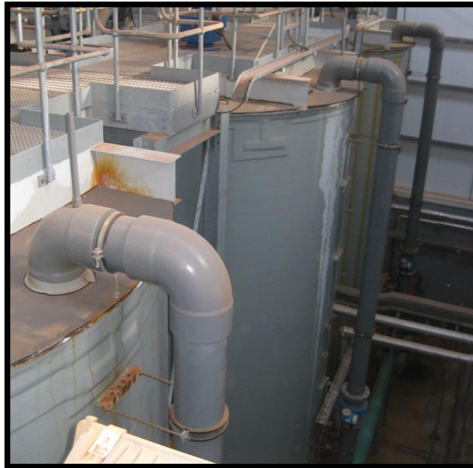
Figure 3-7: 1 st stage reactor tanks for aeration at Dawdon
