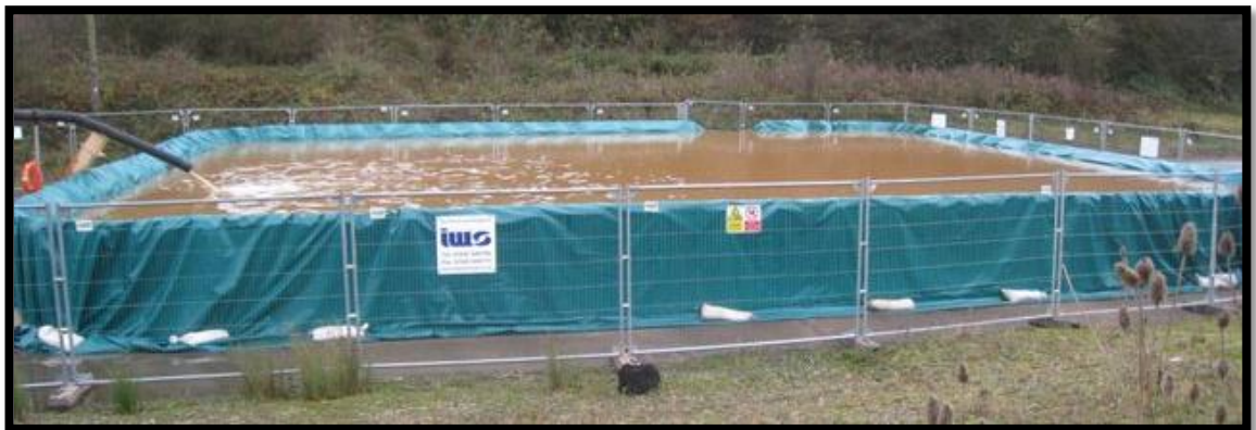
Figure 3-5: Settling pond at Cadley Hill pumping trial
