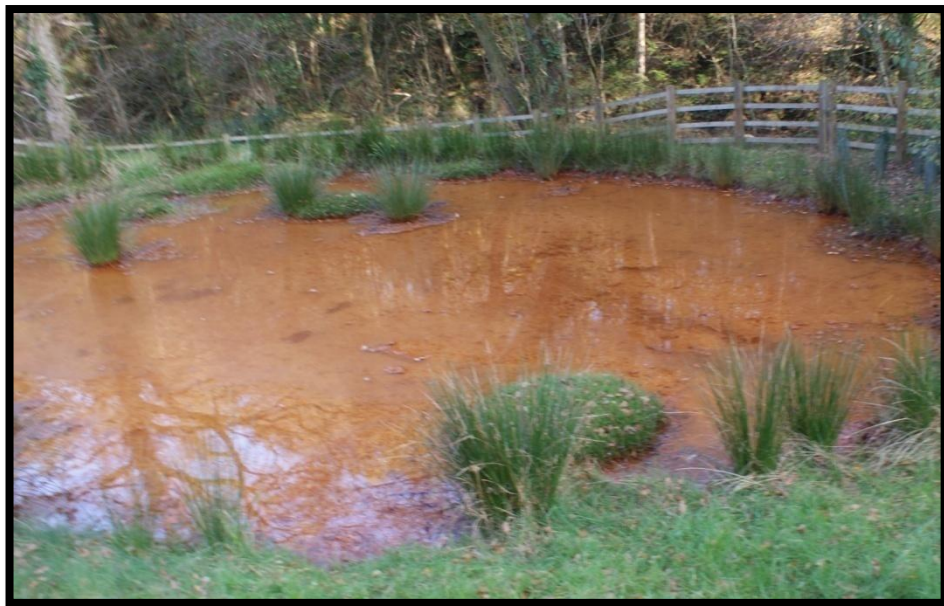
Figure 2-7 Reducing Alkalinity Producing System (RAPS) at Tan-y-Garn, South Wales
