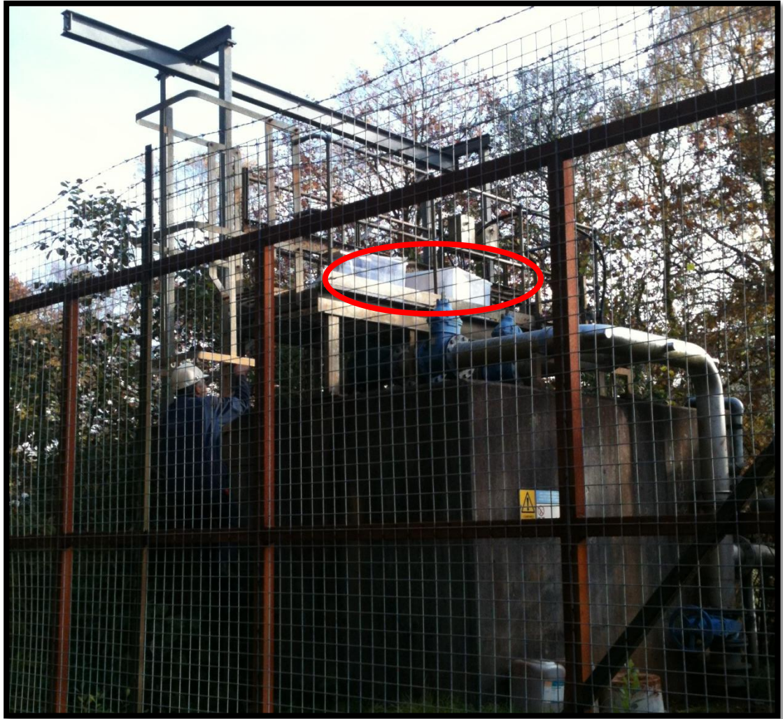
Figure 4-23 Position of continuous flow VFR on top of wet well
