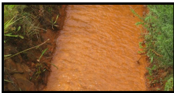
2-1 Distribution channel fouled with HFO precipitates
