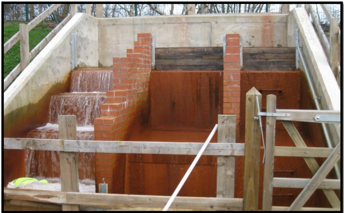
Figure 4-4 Aeration cascades at Strafford (full view)
