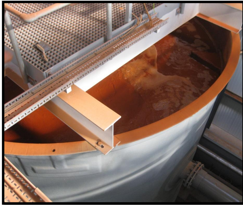
Figure 3-8: Sludge recirculation and lime dosing tank at Dawdon
