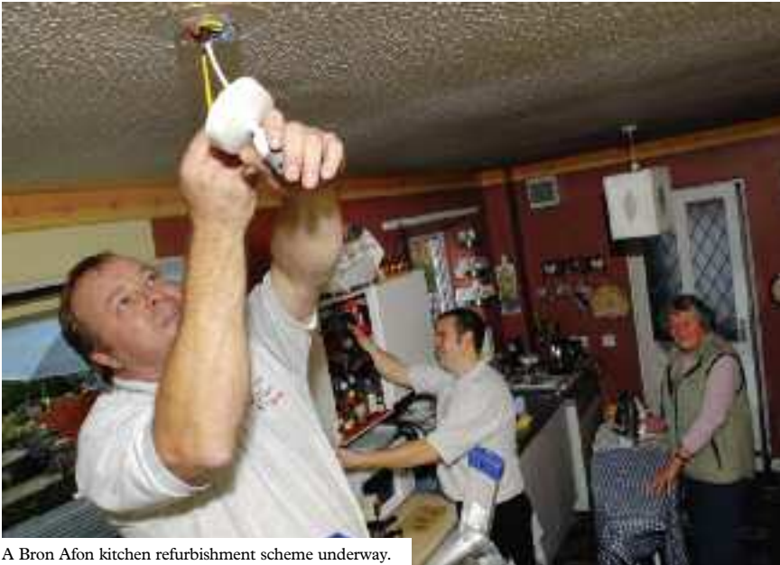
A Bron Afon kitchen refurbishment scheme underway.
