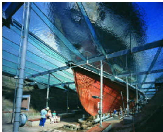
Figure 1 Completed environmentally controlled space for ss Great Britain hull. (Picture courtesy of ss Great Britain Trust and Mandy Reynolds.)
