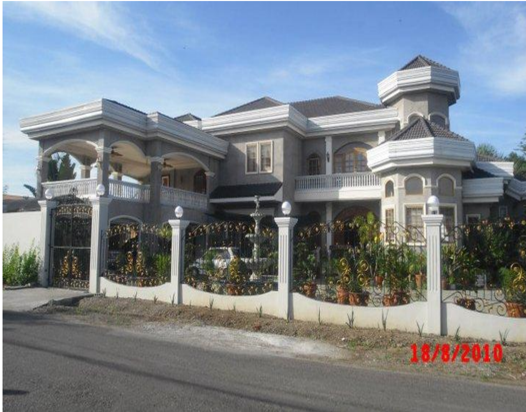
Figure 4.5 The house of a Hawaii/US immigrant. It is popularly referred to as ‘the mansion’. Photo used with permission.
