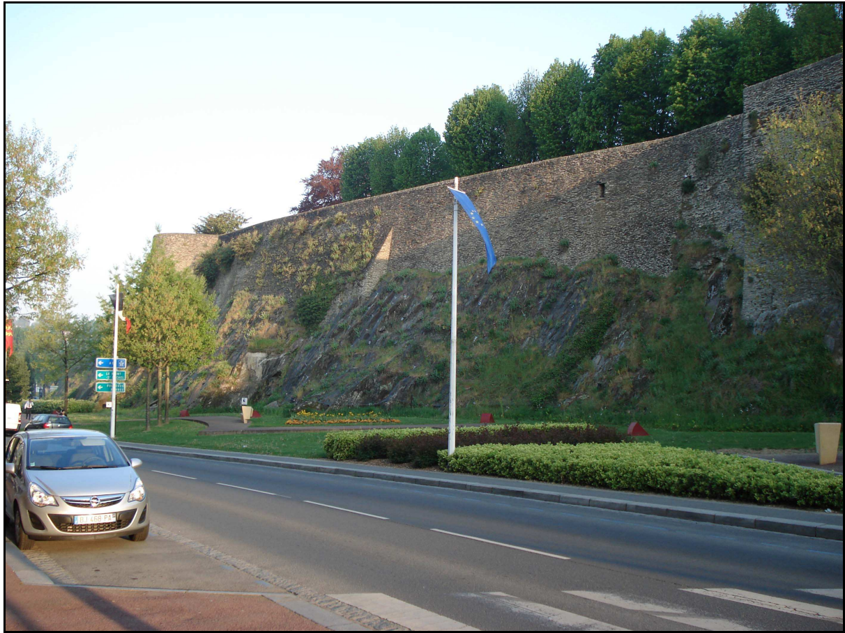
Fig. 9 - Saint-Lô's fortifications, south-west of the church of Notre-Dame: note the bed-rock on which the walls were reconstructed after World War 2.
