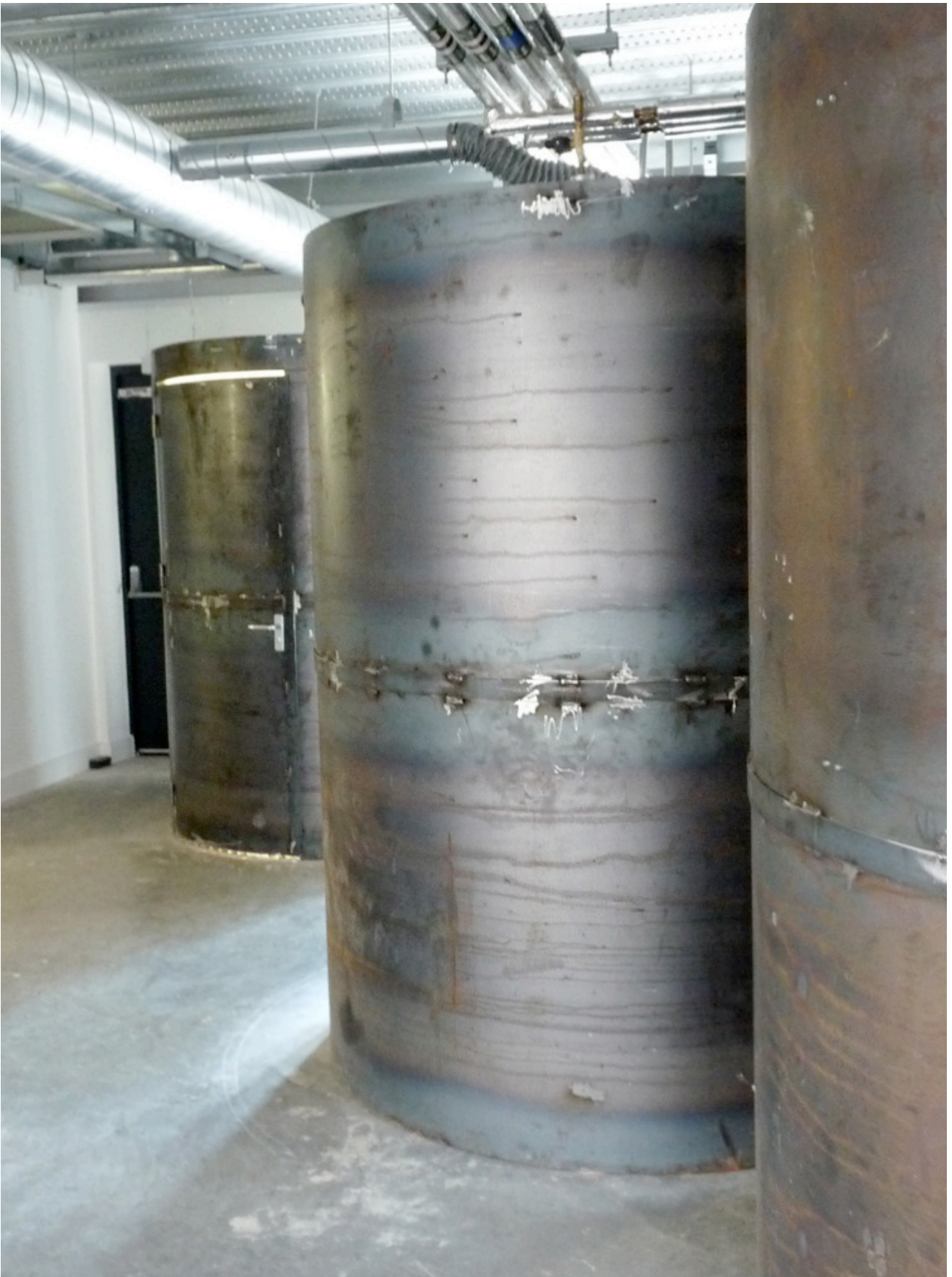
Welfare facilities are installed in steel 'coils'.
