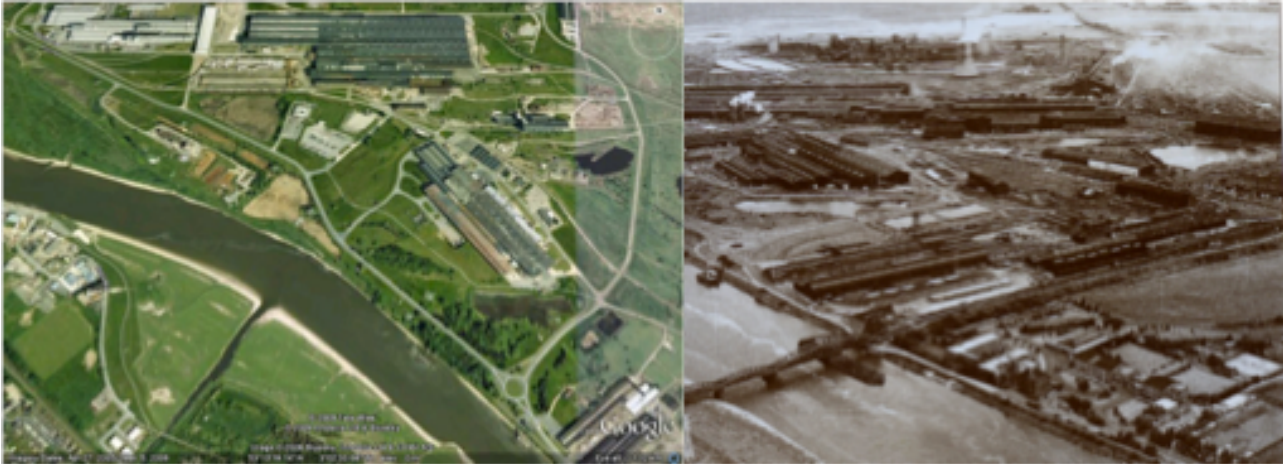
The Shotton site in N Wales – a place of steel making for over 100 years
