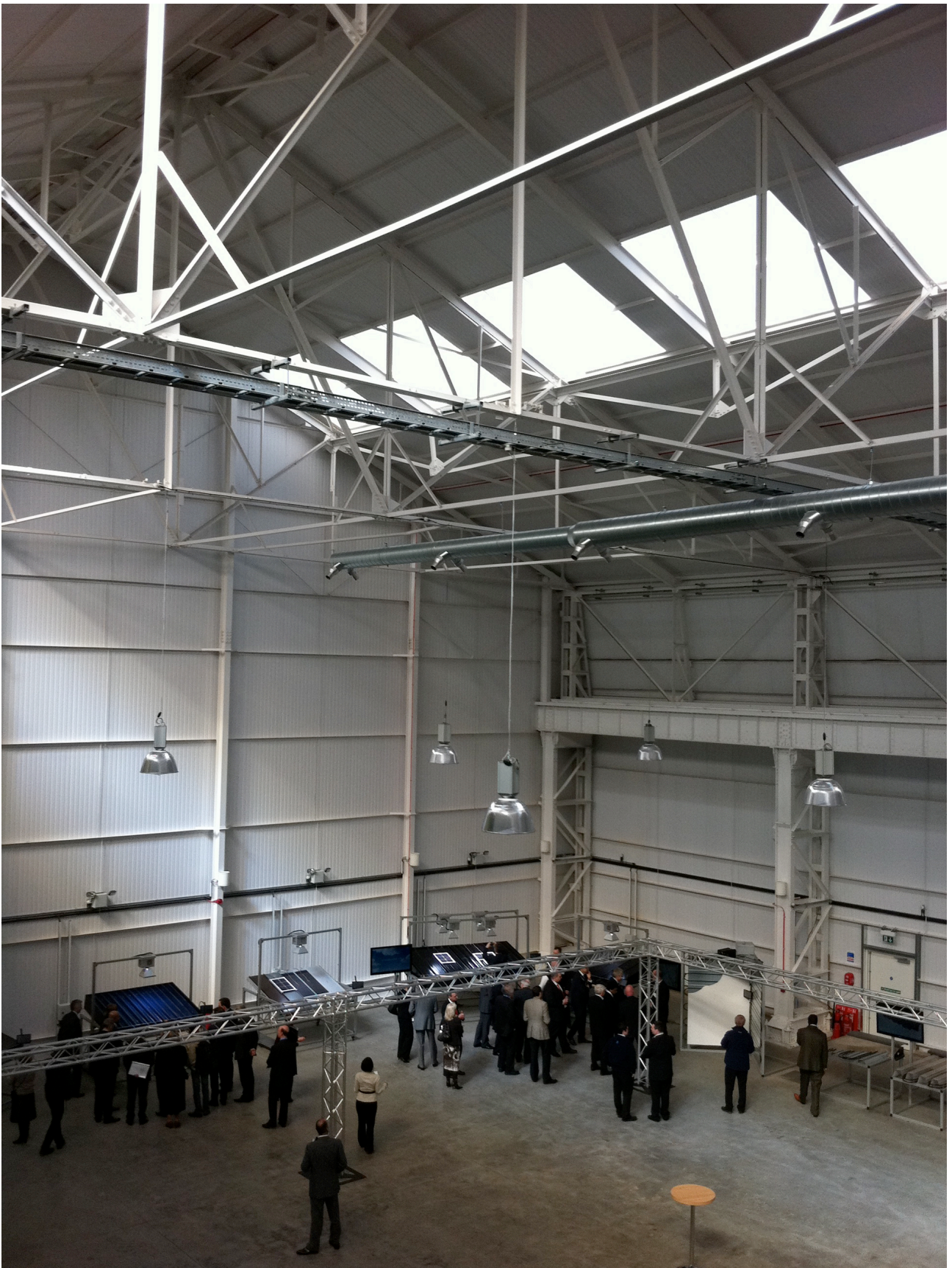
Interior – Note heating duct with delivery nozzles in roof space from transpired solar wall
