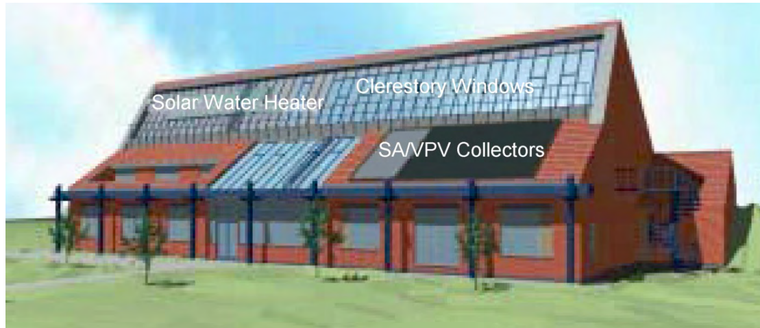
Figure 2.9. Solaf-Luft system on Brocks Hill Millenium Park Environment Centre [14]
