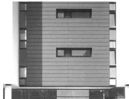
Figure 2.2. Illustration of plank style cladding [9]
