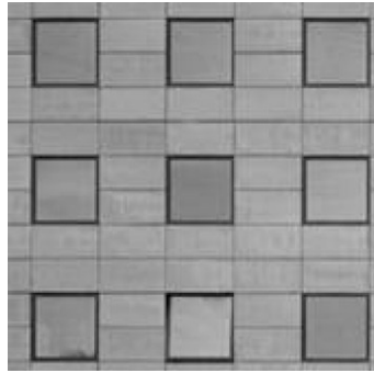
Figure 2.3. Illustration of cassette style cladding [9]
