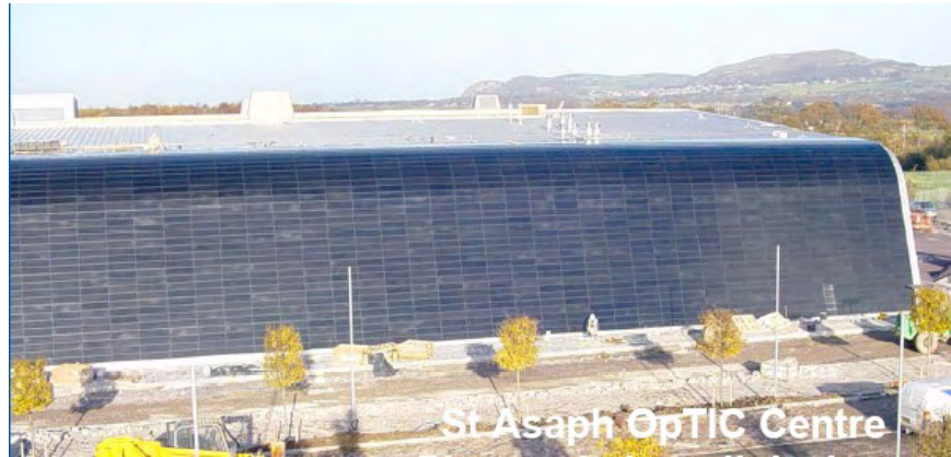
Figure 6.4. St Asaph OpTIC Centre - front view of PV facade
