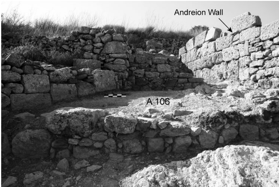
Fig. 4. View of trench A-100 and walls.
