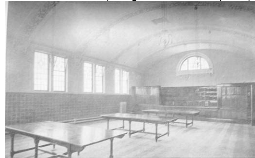
Fig. 8 View: Reference Room 1909 [75]
