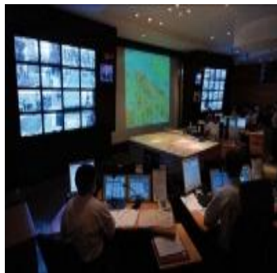
Fig. 12 Central control room Paris
