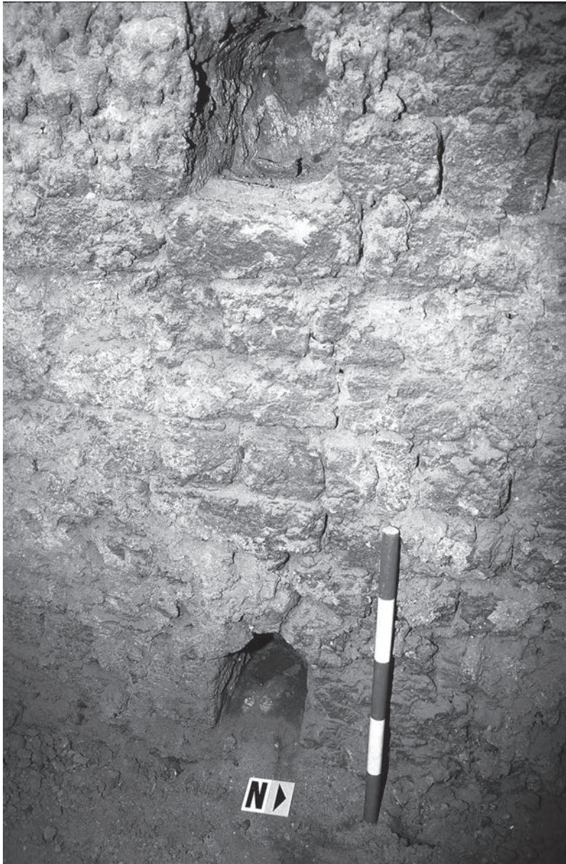
Plate 3.7. Interior view of the west wall of the kiln. The upper vent is [336] and the lower [337]. The upper vent is blocked on the exterior and has a brick wedged into it. The lowermost access opening [235/338] is not yet visible. (Photo: P.T. Nicholson).
