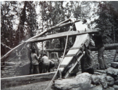
Figure 9.92: Lifting a traditional cruck frame by hand
