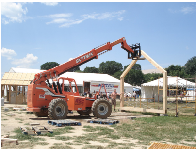
Figure 9.94: Lifting the horizontally assembled portal frame using a forklift onsite for the Welsh Pavilion.
