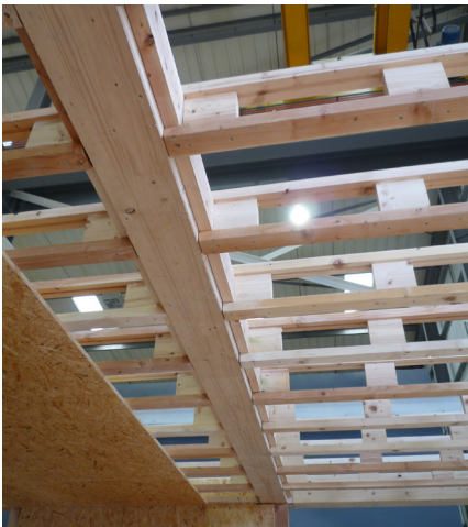
Figure 9.45: Ladder Beam Type 01 employed for the construction of a Ty Unnos Modular unit ceiling, prefabricated into a frame with fixing plate between ladder webs.
