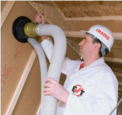
Figure 9.63: Cellulose insulation blown into the closed cavity of a timber frame panel using a purpose made installation hose and nozzle.
