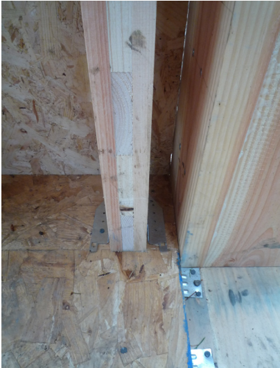
Figure 9.100: Access to face fixed joist hanger fixing points is extremely limited when adjacent to primary structure.
