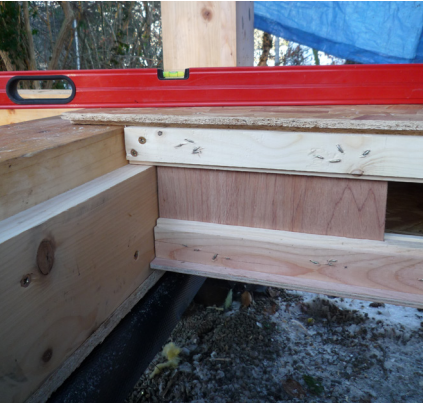
Figure 9.101: Installation of infill panels to Bay 2 day 1
