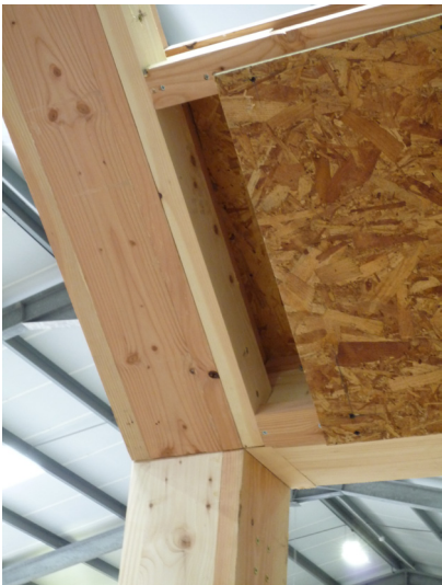
Figure 8.69: Prefabricated infill panels awaiting installation with notched ladder beam and external OSB sheathing.
