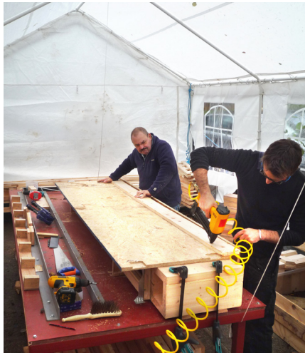
d) A precut and routed OSB sheathing is prepared with a spruce board nailed to the long edge to provide connection with neighbouring panels.
