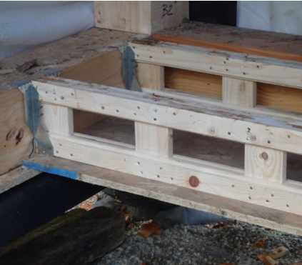
Figure 9.98: Installation of infill panels to Bay 1 day 1
