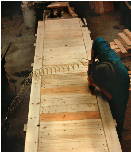
f) Lateral spruce boards are double nailed to the ladder flange.
