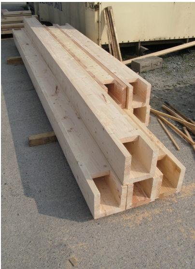
Figure 8.65: Assembling bolt laminated angled connectors for the eaves junction of the primary portal frames. Figure 8.66: Bolt laminated connectors. Figure 8.67: Ground floor box section beams with notched ends to receive connectors.
