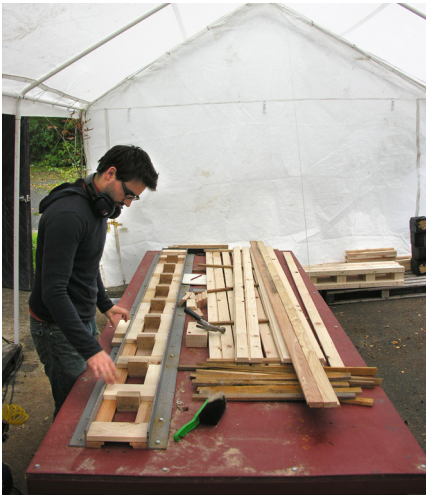
d) Insert boom infill timbers between webs, the first web spacing is reduced to set out the remaining webs at 300mm centres.
