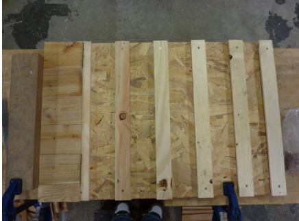
a) 25x50mm pressure treated softwood horizontal battens are set out at even centres.
