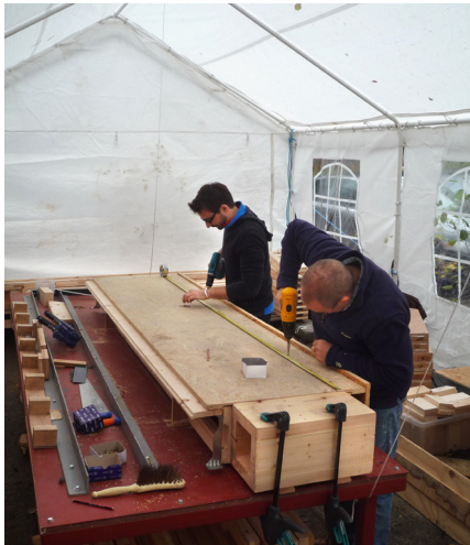
f) Screws are installed at equal centres through the sheathing into the ladder boom.
