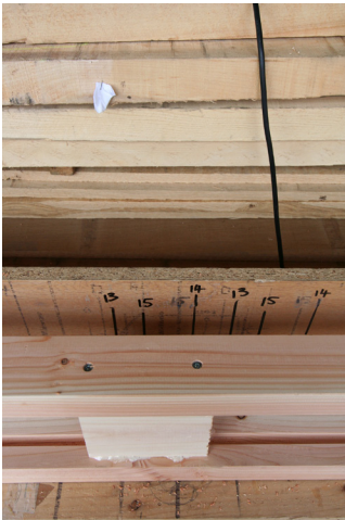
c) A setting out template is marked up with standard web and screw centres to assist assembly.
