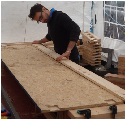
Figure 9.54: 18mm OSB sheathing panel routed to a depth of 9mm to recieve oversized joist hangers.
