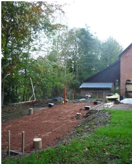
c) Site is levelled and cleared and a layer of sand laid across the site.
