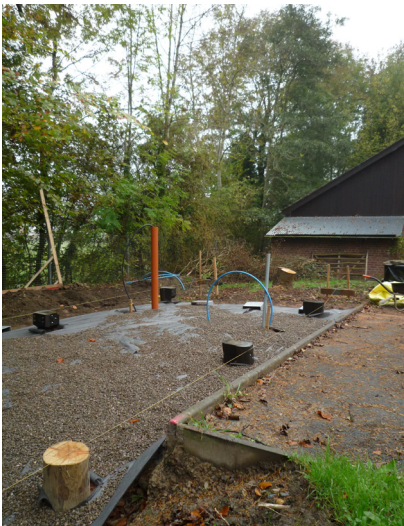
d) A heavy duty weed barrier membrane is cut and fitted around services and piles and weighted with pea shingle.
