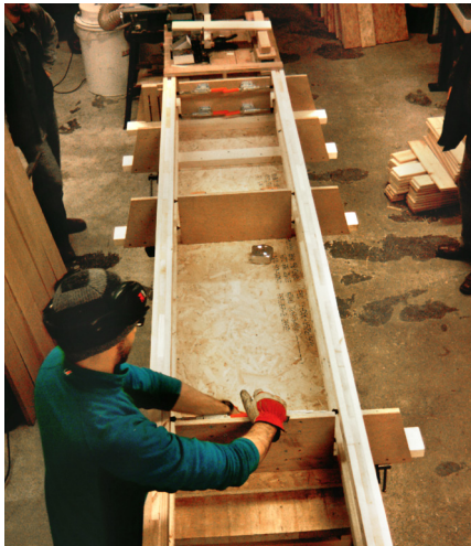
c) With ladders in place, push clamps fixed to fins push ladders tight against the plywood retainers ensuring a parallel fixed width.
