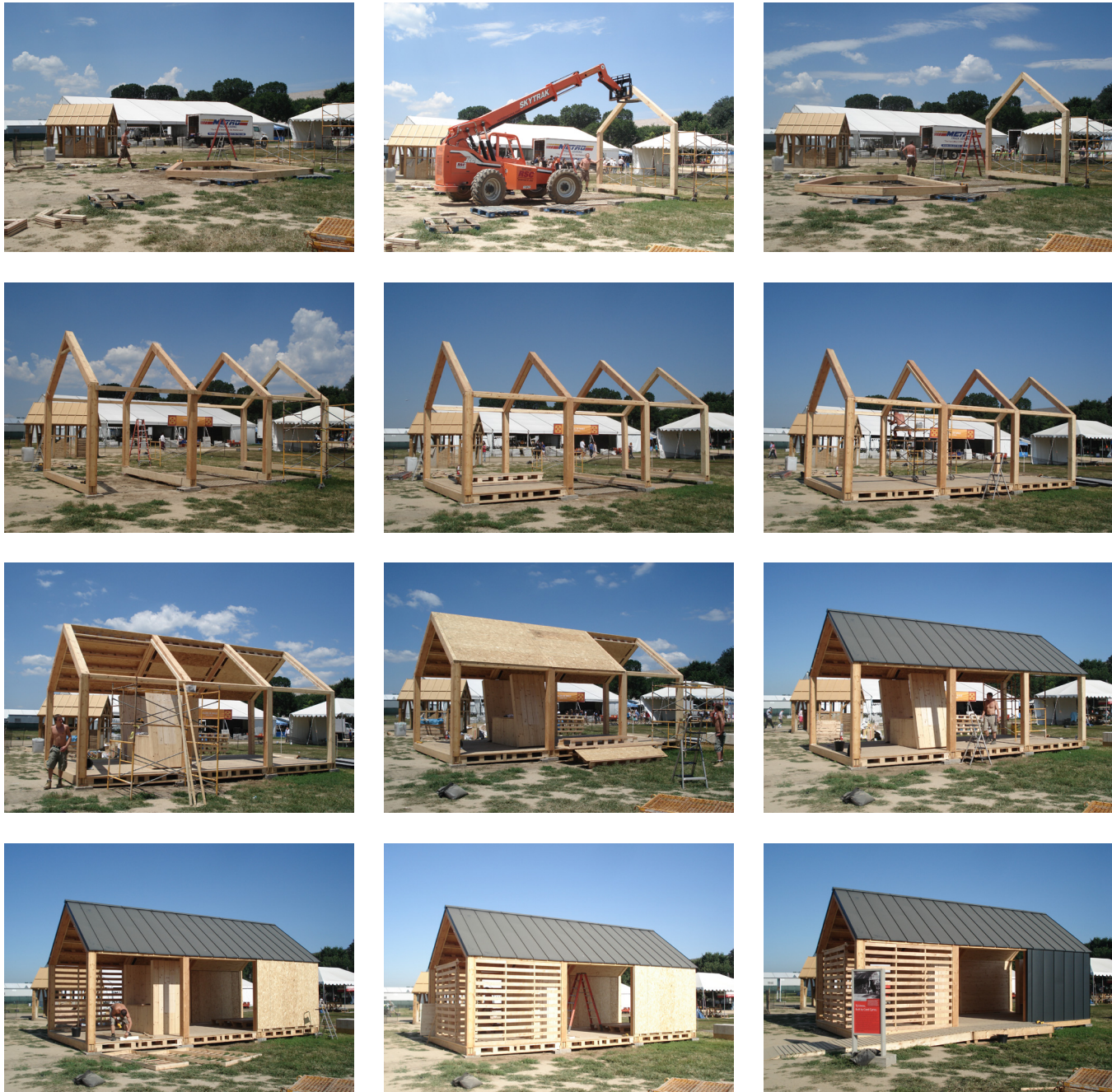
Figure 8.68: Construction sequence on the Washington Mall
