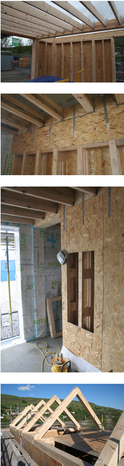
Figure 8.98: Intermediary floor joists installed on joist hangers face fixed directly to floor beam. Figure 8.99: Metal straps across intermediary floor zone to connect diaphragm panels. Figure 8.100: Living room internal wall with viewing panel to ladder beams. Figure 8.101: Intermediary floor installed at loft level with roof trusses awaiting roof infill panels.
