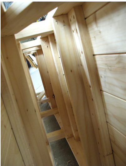
Figure 6.56: Sitka spruce based panel prototype combining internal and external sheathing of T+G with spruce ladders. Figure 6.57: OSB based panel prototype including air tightness seals. Figure 6.58: Interior of spruce based panel showing substructure of additional noggins .
