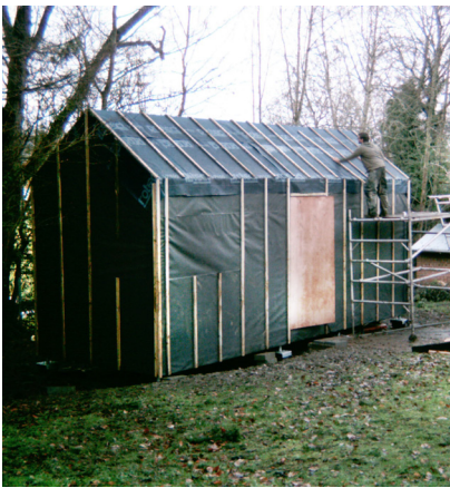
d) Apply 25x50mm pressure treated softwood vertical battens
