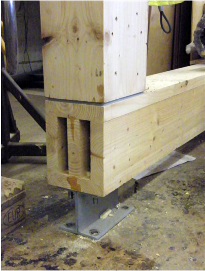
Figure 9.26: Hot rolled steel I section foundation footing as used for the Ebbw Vale Resource Centre including steel bearing plate between beam and column.
