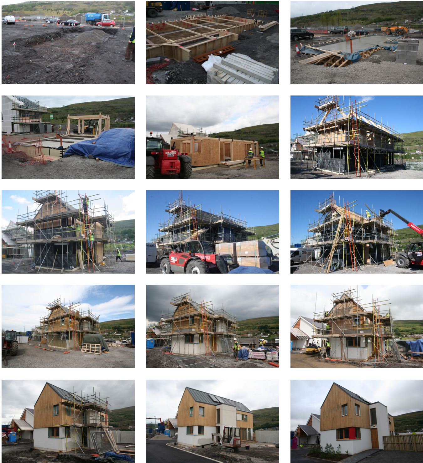
Figure 8.97: Construction sequence of the Passive House.
