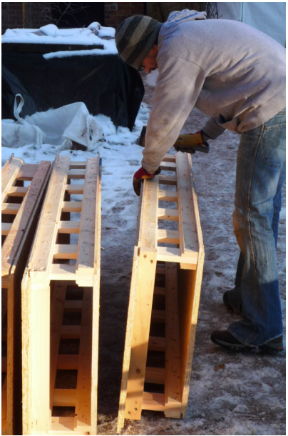
Figure 9.86: 9mm plywood tongues are inserted as a final operation immediately prior to installation on site.
