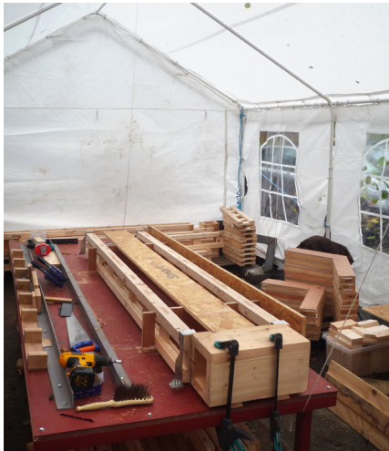
c) Box section stop ensures ladders are set square to the OSB side rail.
