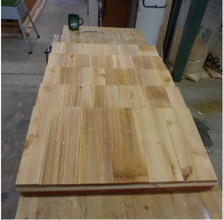
d) Shingles require a level of selection to maintain a reasonable consistent thickness to the exposed edge.
