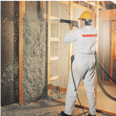
Figure 9.62: Damp cellulose insulation blown into an open timber frame panel
