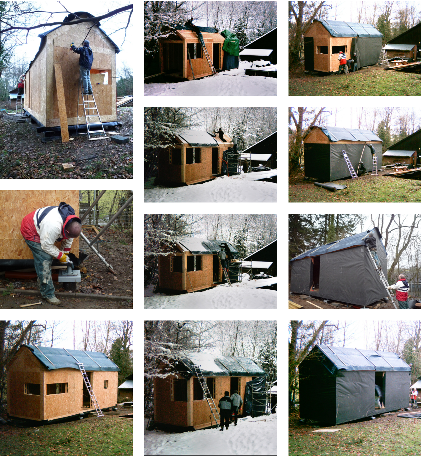
a) Prepare external skin for breather membrane
