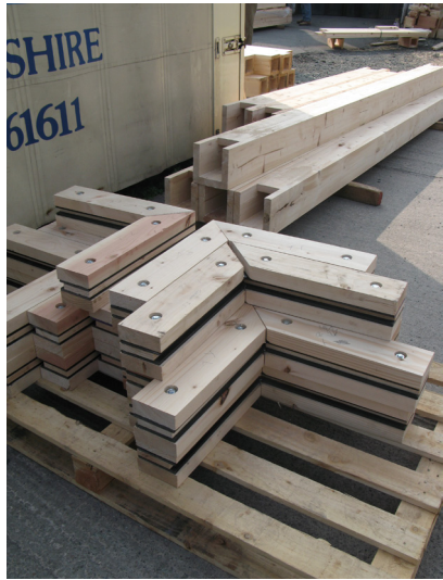
Figure 9.35: Steel and softwood hybrid bolt laminated connectors, left over from the construction of the Welsh Smithsonian Pavilion.
