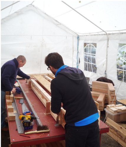
b) Place a second ladder into location. Plywood fins ensure ladders are set parallel and accurately centred.
