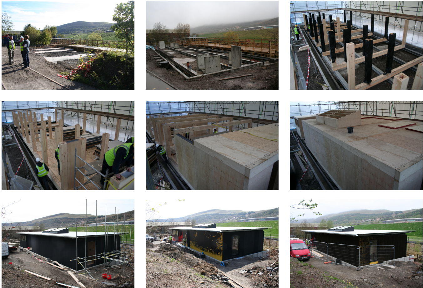
Figure 8.44: Construction sequence of the ERC.
