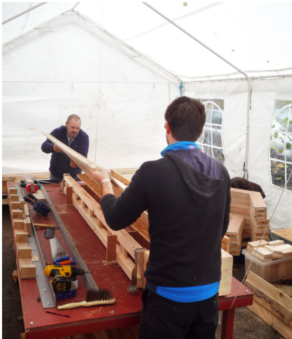
e) Sheathing is turned over and positioned on ladders with routed grooves located over the oversized joist hangers.
