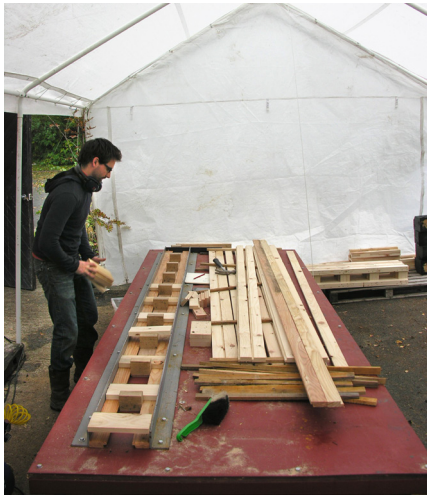
c) Insert web timbers into the jig and tap down flat against boom timbers, oak spacers act as a guide to web spacings and right angle.
