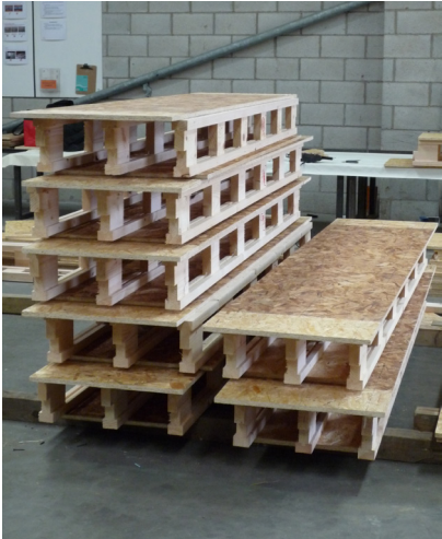
Figure 9.57: Infill panels with notched ladder beam detail awaiting assembly for the Welsh Pavilion.
