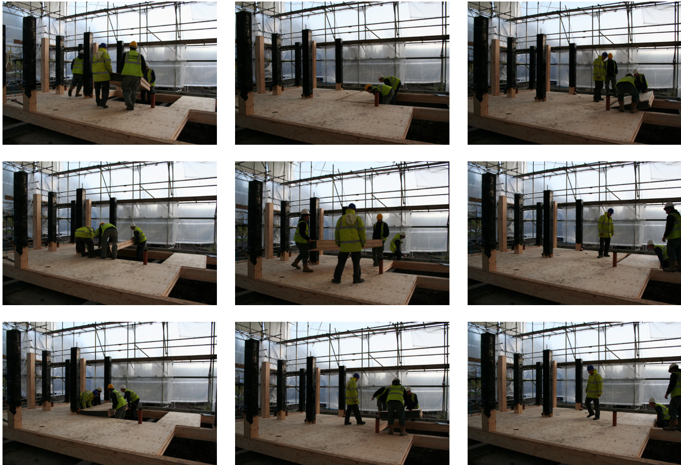
Figure 8.35: Floor infill assembly sequence FROM TOP LEFT ACROSS - DOWN
