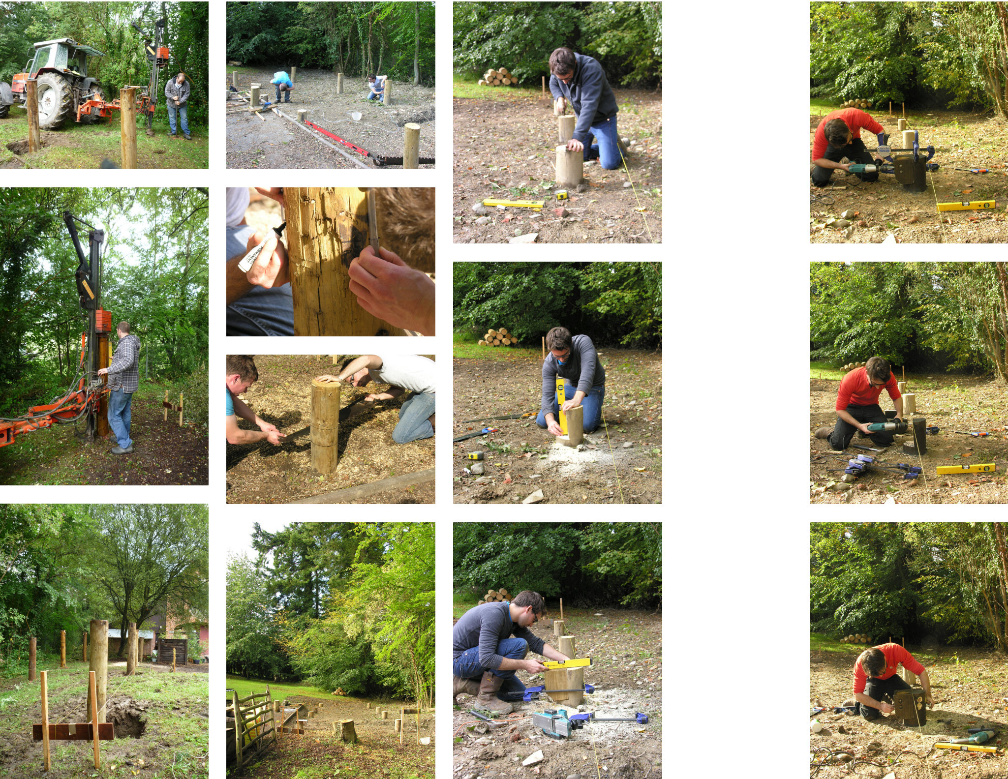
Figure 9.89: Installation and preparation of timber piles to receive primary structure
