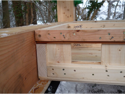
Figure 9.102: Installation of infill panels to Bay 3 day 1
