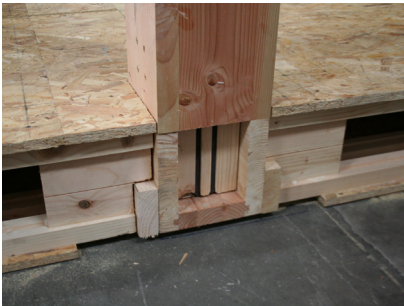
Figure 9.56: Notched ladder beam and timber bearing plate detail employed for the Welsh Pavilion.
