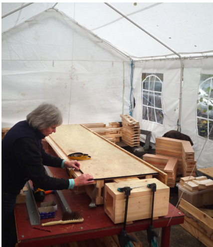
h) An adhesive seal is applied to the perimeter of the panel intended to compress against neighbouring panels and structure to improve airtightness.
