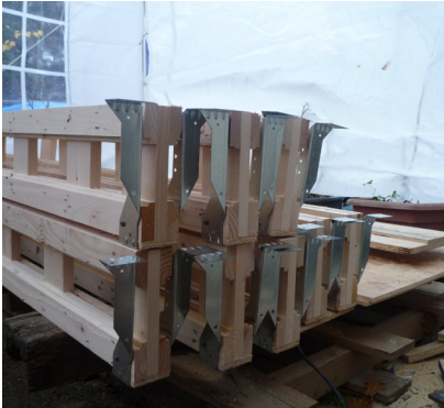
Figure 9.99: Manufactured ladders with top hung joist hangers fixed into bottom boom, with 9mm OSB packing piece to increase depth.
