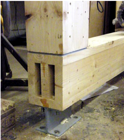
Figure 6.33: Threaded rod connection manufactured by Cowley Timberwork showing spreader plate, foundation connection and additional compression timber.
