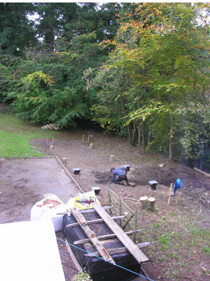
a) Site levelled using a mini digger and adjacent sycamore tree removed. A service trench is prepared from Bay 1 to the existing sanitary facilities in the Old Sawmill.
