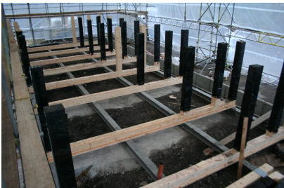
Figure 8.31: Box section lamination press. Figure 8.32: 7.2m box beams prepared with additional supporting timbers installed to floor beams Figure 8.33: Threaded rod connection detail with spreader plate and rolled I section foundation connector. Figure 8.34: Floor beams and columns installed on site.
