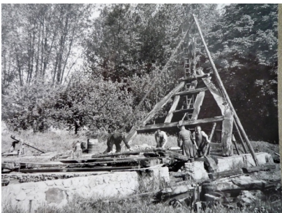
Figure 9.93: Lifting a traditional cruck frame with the assistance of a triangular truss
