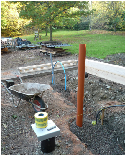
b) Cold water supply, armoured electrical cable and waste pipe laid into trench on sand base. Safety tape laid above electrical cable and trench infilled with layer of sand and pea shingle.
