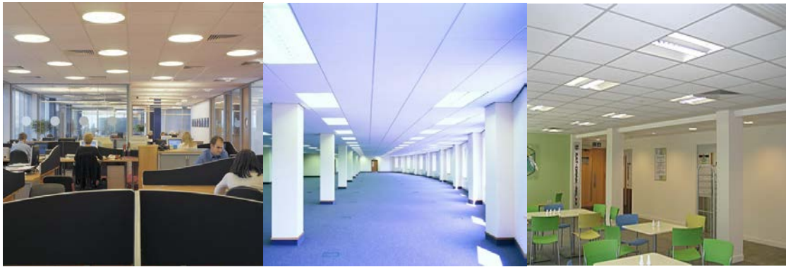
Figure 2.2 Examples of ceiling luminaires placed at regular intervals
