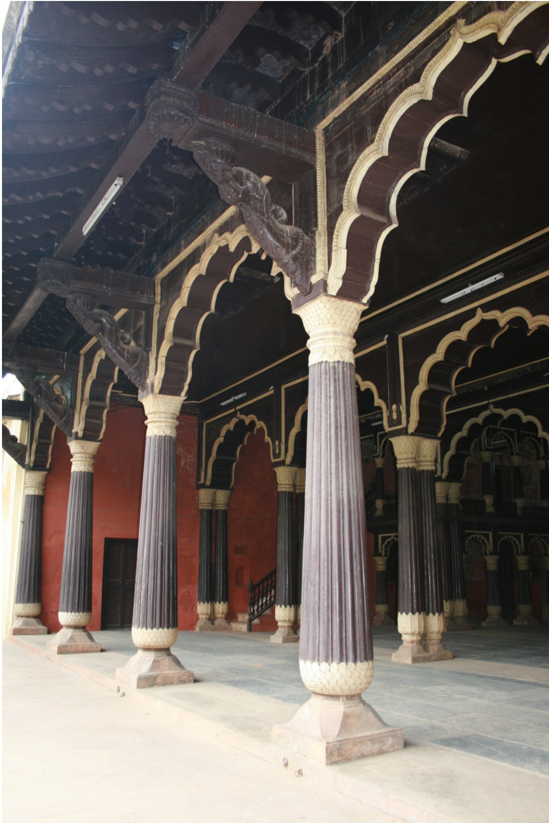
Fig. 3.4.19 Overhang supported by elephant brackets
