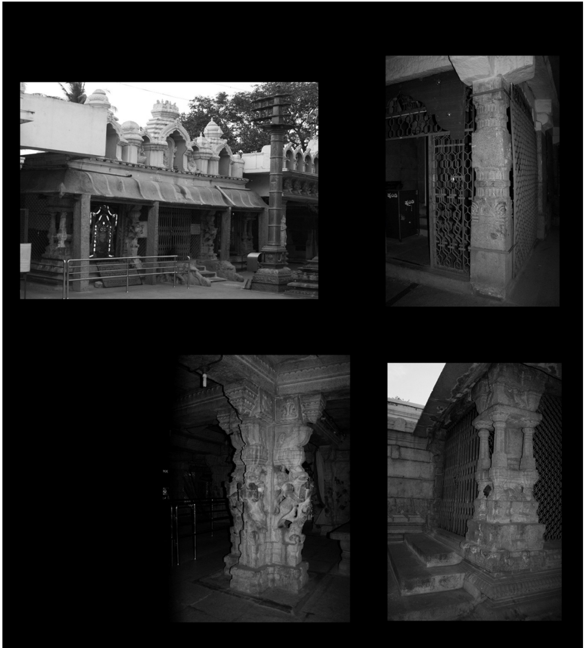
Fig. 3.1.9 Venkaṭaramaṇa Swāmy Temple near Oval Fort, K R Road – Images showing basic and composite columns with colonettes on three corners and figural additions on all four sides
