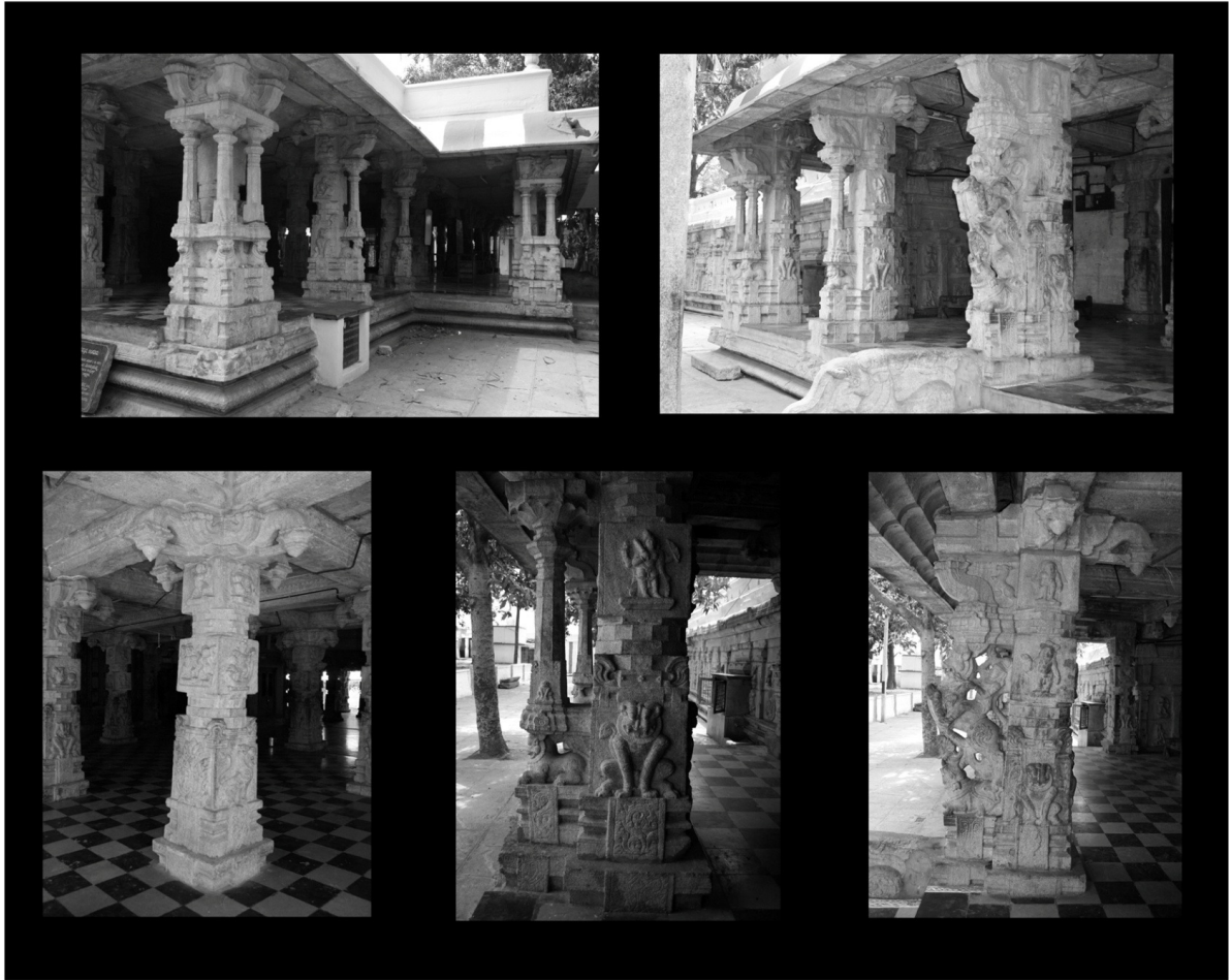
Fig. 3.1.12 Halasūr Sōmēshwara temple – Images show basic and composite columns - single and three corners colonette, and single figural columns
