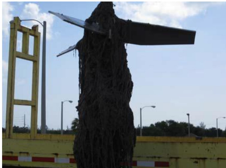
Figure 10.12: - Ragging on an impeller within a municipal wastewater treatment plant taken from Glass (2010).
