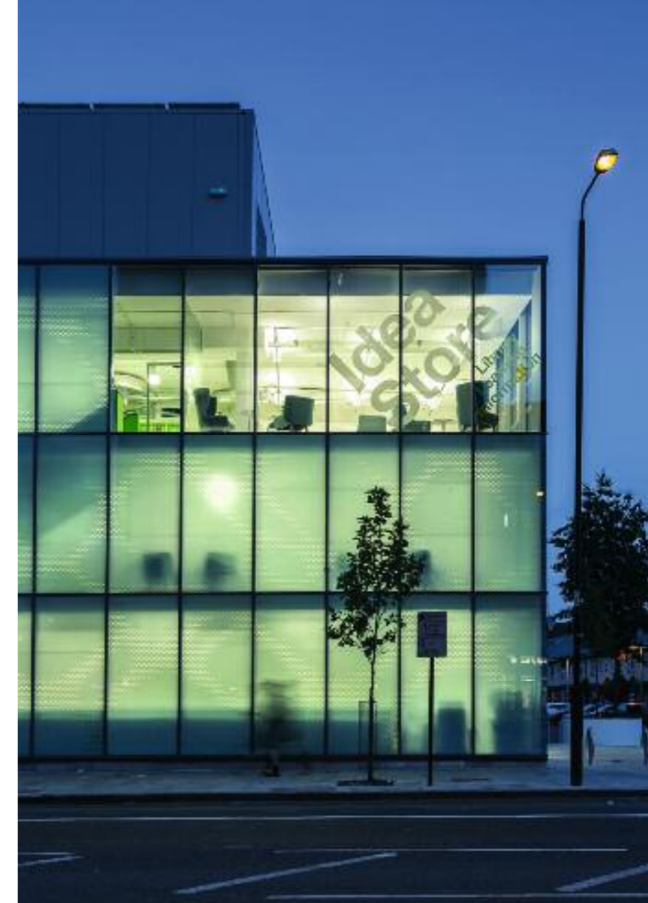
Right The facades comprise four glass layers with two cavities. Below Cross section; north-west corner window with signage.
