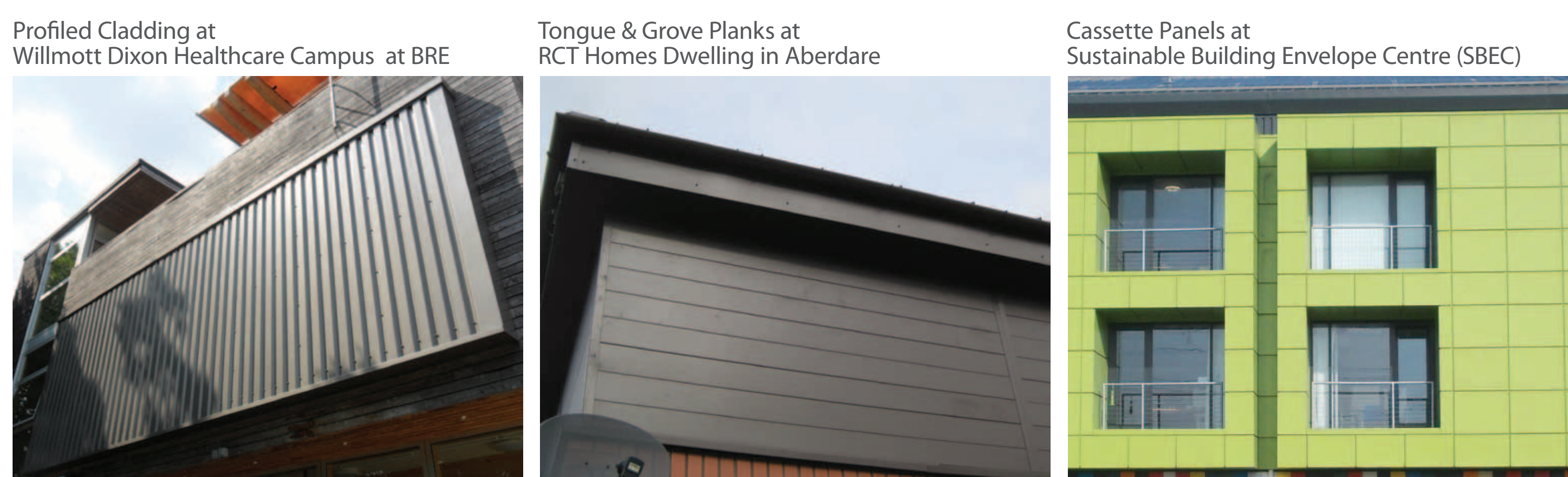
Fig. 4. Examples of the three different types of metal cladding available for Transpired Solar Collectors
