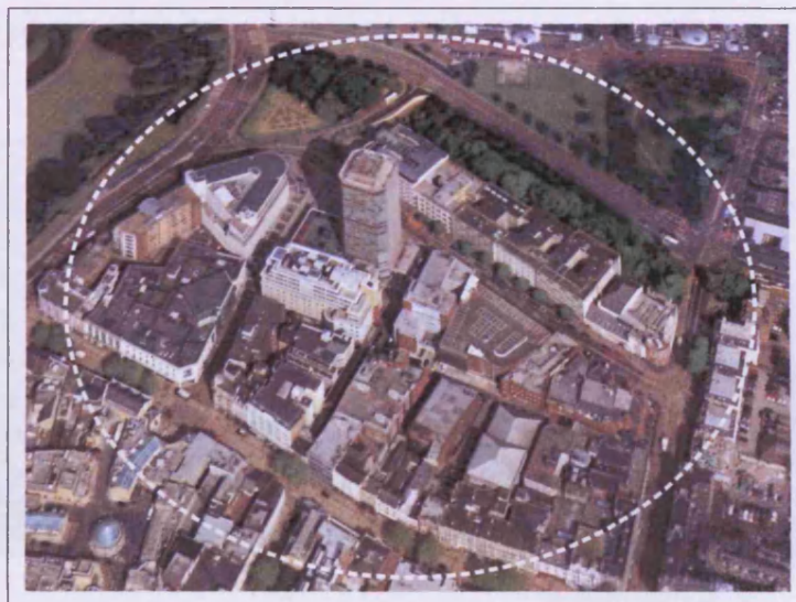
Figure 55: Aerial photograph of site showing perimeter of case study area 286
