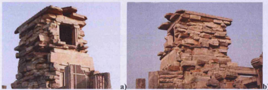
Figure 156: a) & b) Temple 45, views of the rough core of the śikhara .
