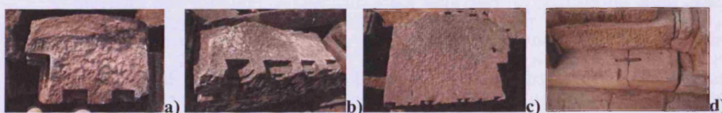
Figure 149: a) SAN 249, pratilatā course b) latā course c) SAN 359, pratilatā course d) Blocks of stone 'stapled' together in front of the doorway of the Jarāi-kā-maṭh at Barwasagar.
