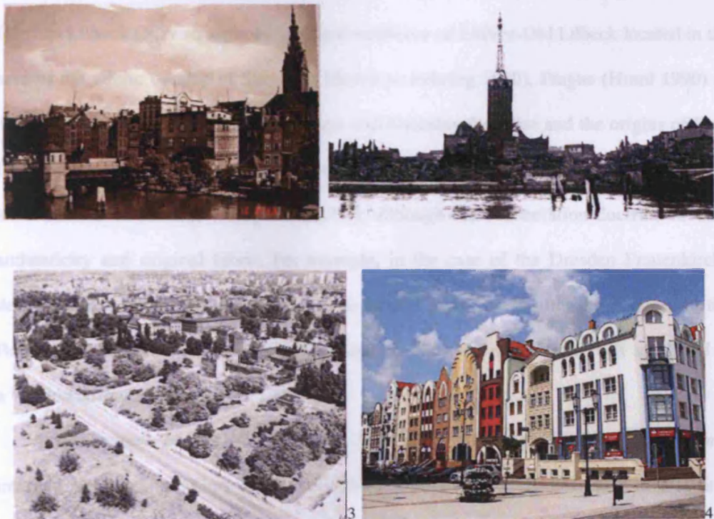
Figure 25: Elbląg Old Town: 1-2 – Old Town panorama in 1943 and in 1945; 3 – Demolished Old Town converted into a green open space in the post-war period; 4 – 1990s redevelopment on medieval foundations (source: www.elblag.eu ).
