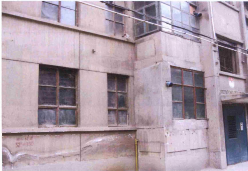
Figure 7.8: Out-dated Building Construction. Source: Author
