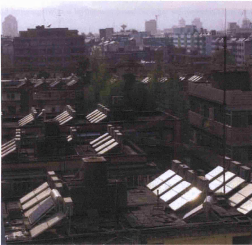
Figure 7.24: Solar Water Heating System in China. Source: (Steffen 2006)
