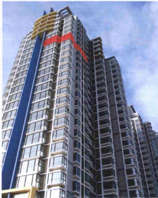
Figure 5. 39: Facade of Third Case Study Flat, Building No. 6
