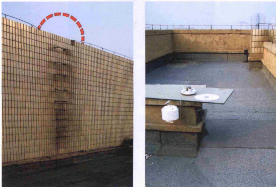
Figure 5. 9: Loggers were placed on top of the building
