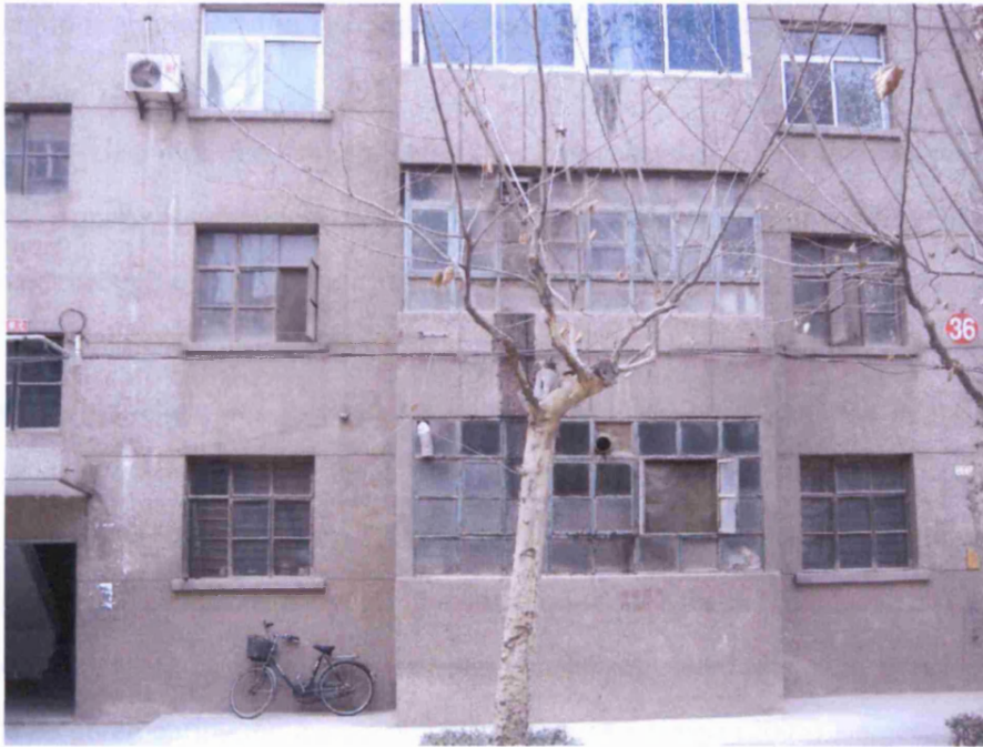
Figure 7.18: Out-dated Housing in 80's in Xi'an. Source: Author
