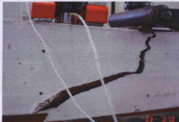
Figure 4.50: Beam C11PS at failure.
