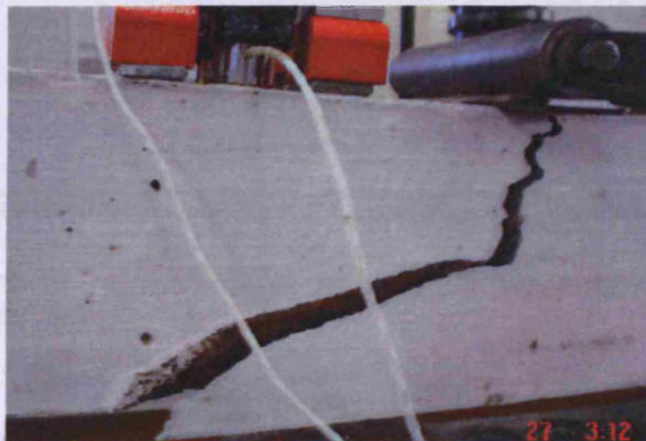
Figure 4.50: Beam C11PS at failure.
