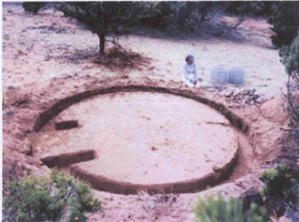
Figure 3.3 Step two the perimeter was trench dug out
