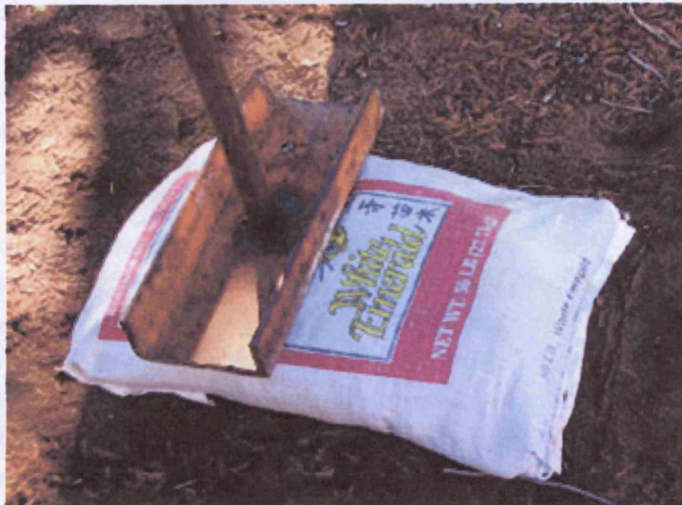
Fig.3.5 Step four: Filling of bags with soil
