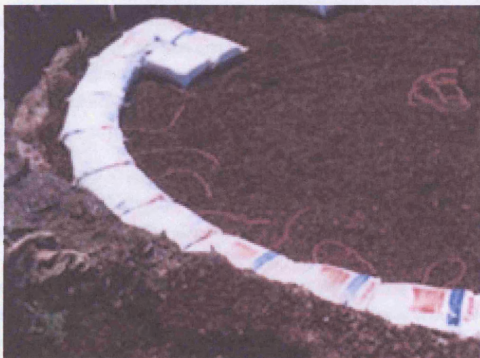
Figure 3.6 laying bags in the trench
