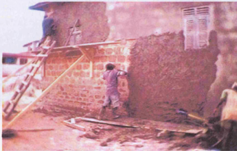
Figure 2.1 Rehabilitation of sunburnt house using aktagbame method of construction
