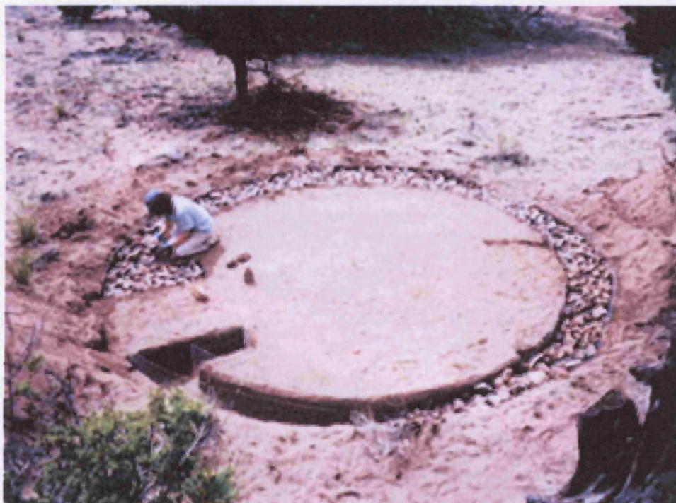
Figure 3.4 Step three: the trenched was filled with rubble
