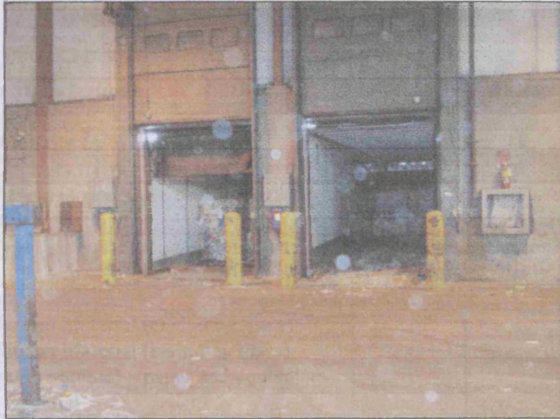
Figure 4.10: Trailer loading Bays at Guelph Wet Dry+ MRF
