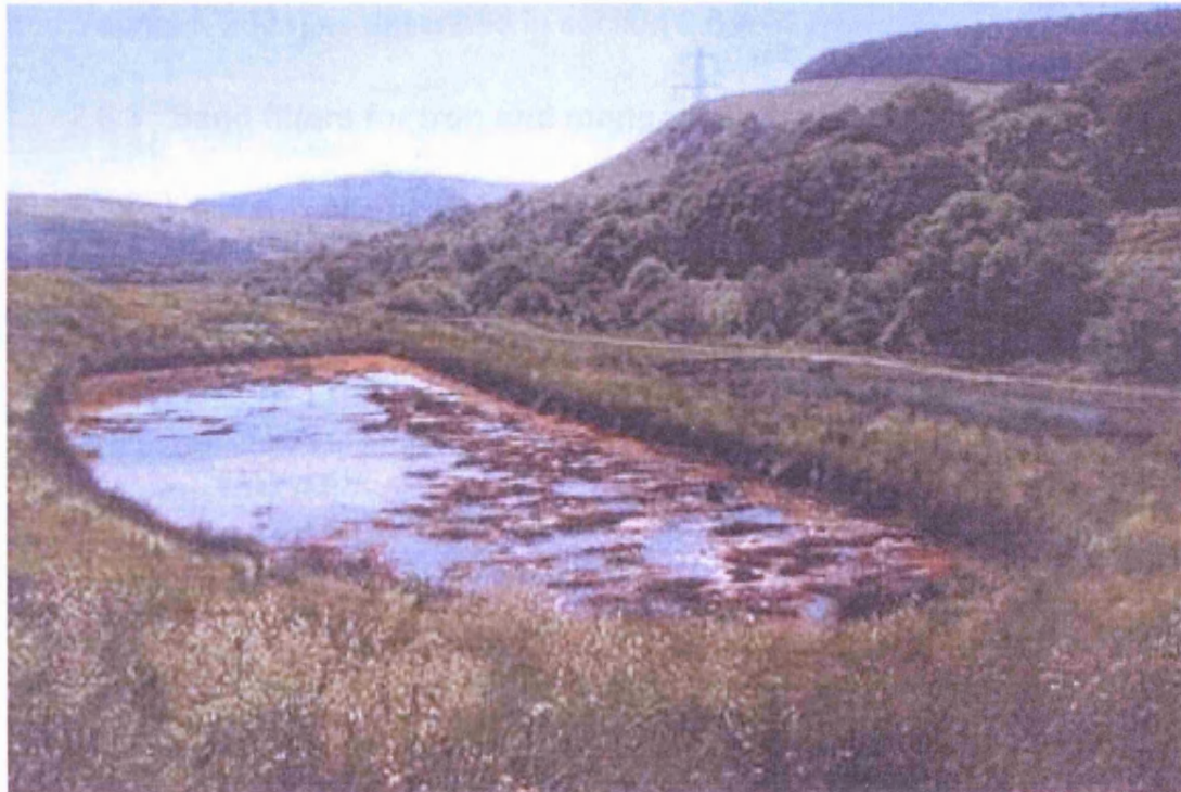
Figure 2-5: Whitworth A RAPS system showing ochre precipitation on compost surface
