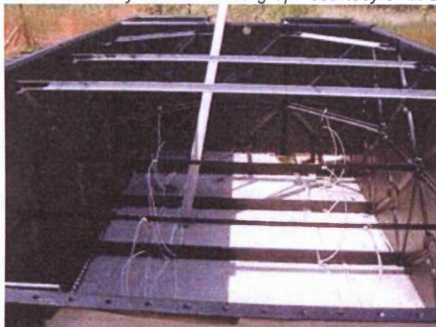
Figure 4-15: View facing west of the inside of the sectional steel tank (looking towards the discharge end) The wooden struts, sample tubes, steel cross members and the gap below the baffle wall can be seen. Photograph courtesy of Dr Devin Sapsford.
