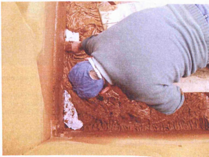
Figure 4-25: Using cotton rags to block short-circuiting pathways around the tank walls
