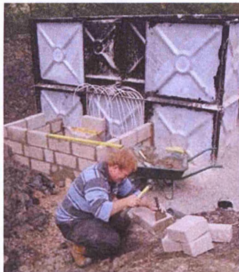
Figure 4-21: Construction of the discharge chamber.
