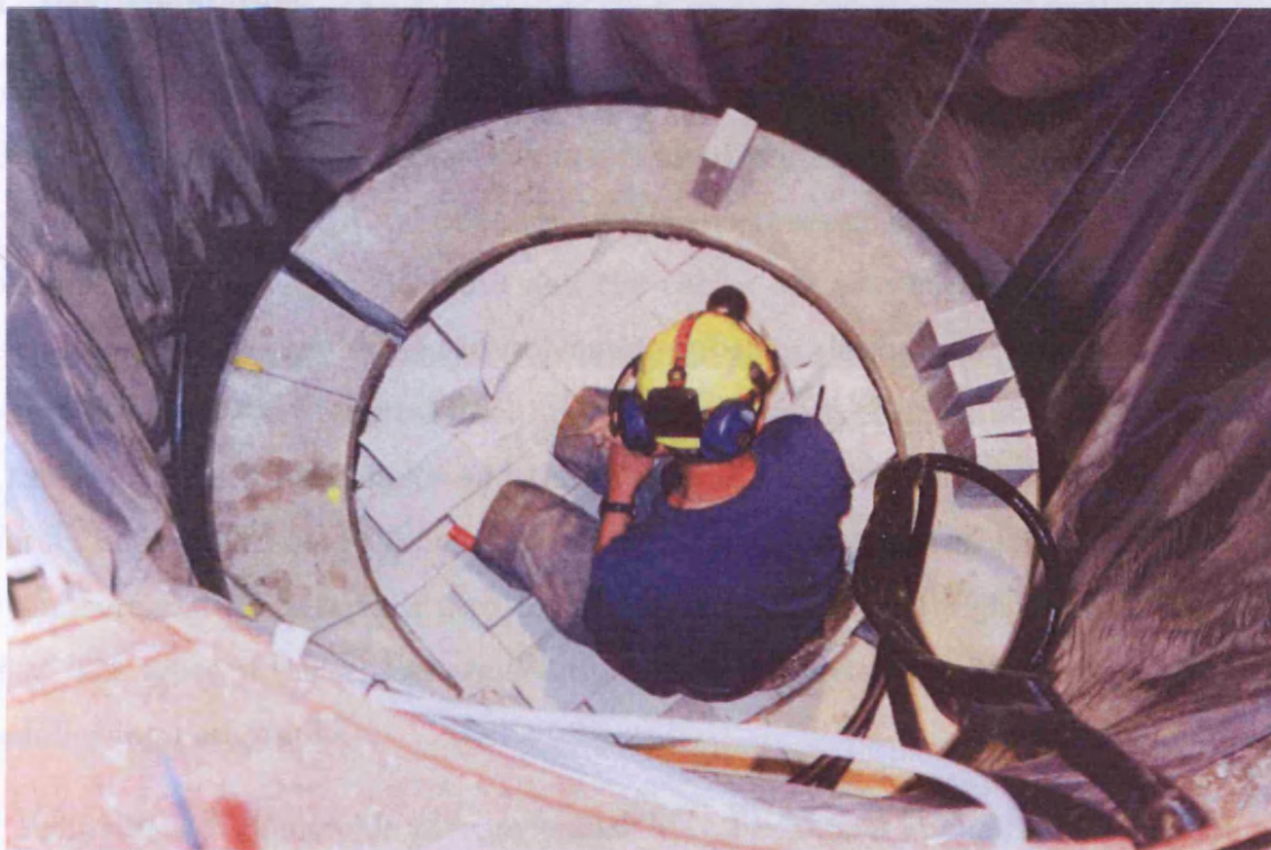
Figure 6.15. Installation of the bentonite bricks on the top of the canister (Johannesson et al. , 2004).
