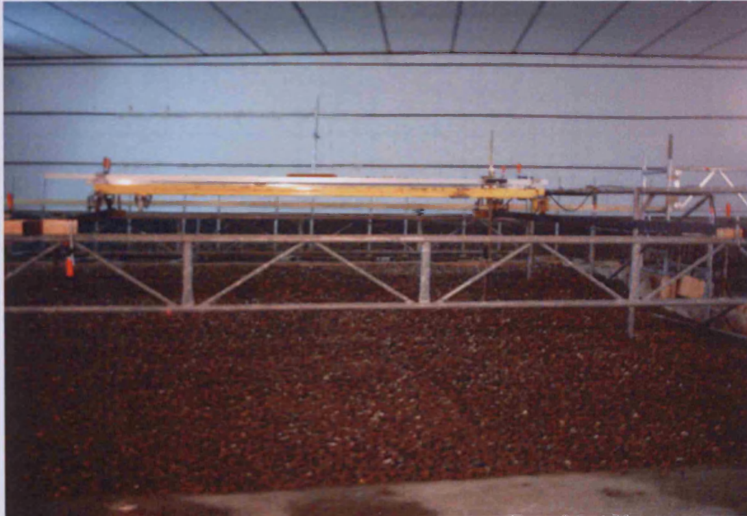
Figure A1- 10. The additional structure
