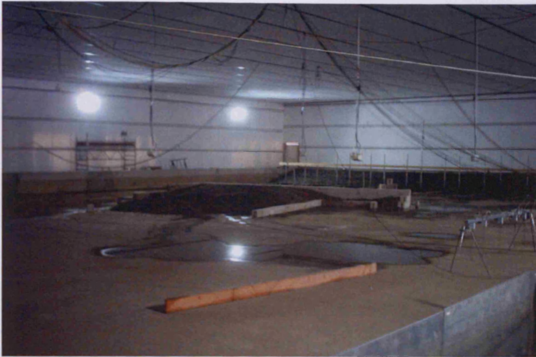
Figure A1- 3. First stage of construction
