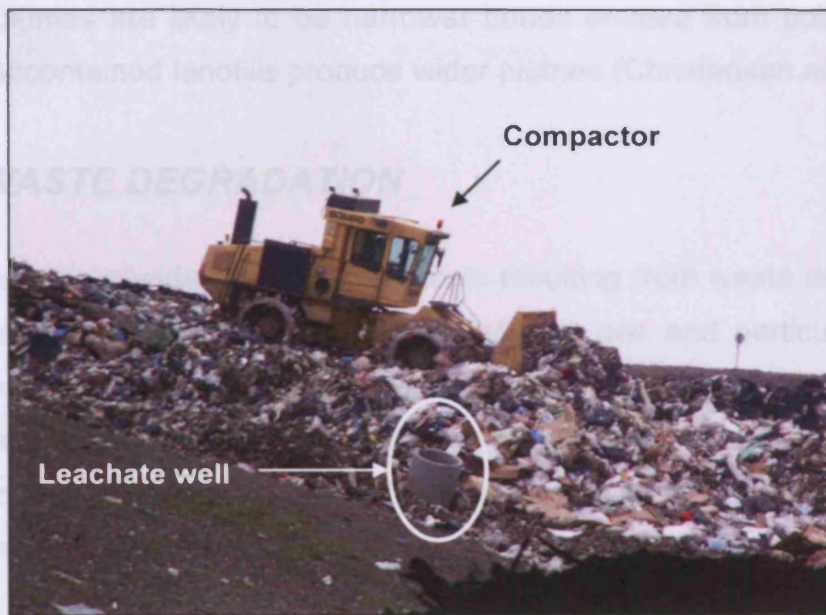
Figure 1.5: Waste compaction and leachate well in a modern landfill. Image by L. Koshy.
