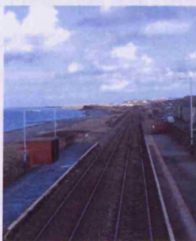
Workington, Network Rail
