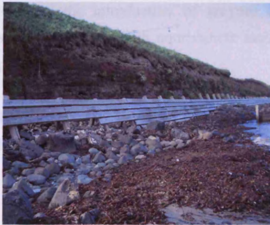
Retaining wall (western section of bay)
