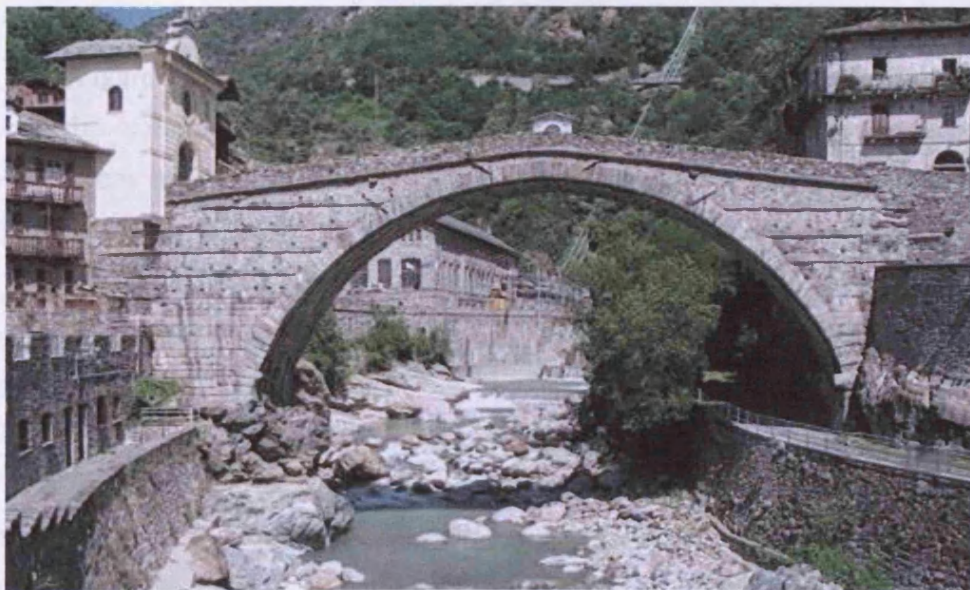
Figure 5.1 Example of bridge data from photo Pont-Saint-Martin
