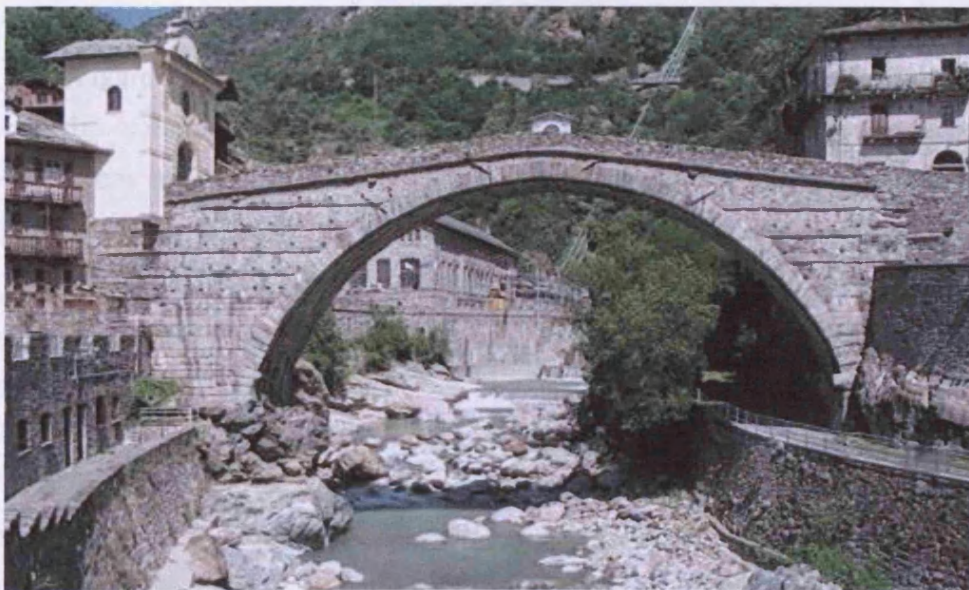
Figure 5.1 Example of bridge data from photo Pont-Saint-Martin
