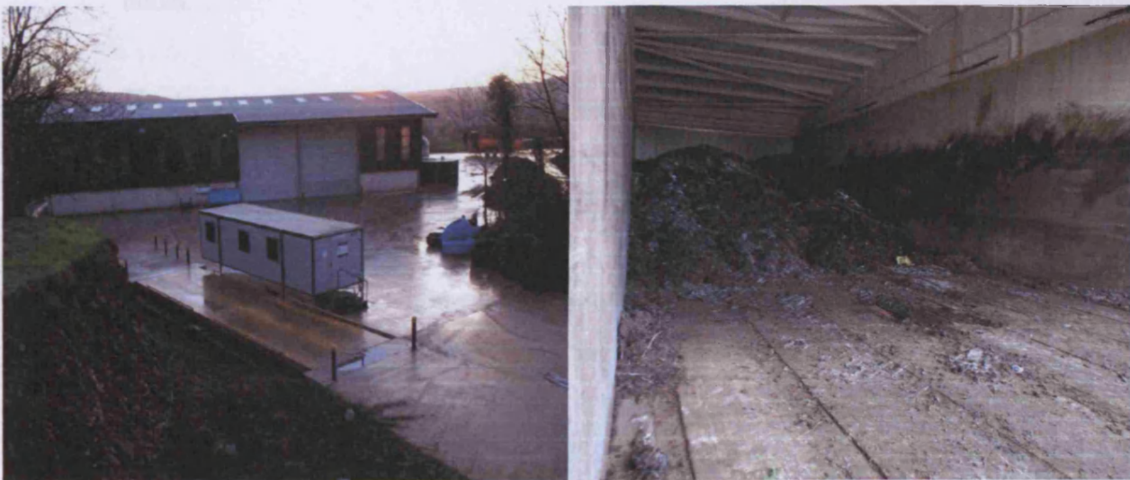
Figure 6.45 Bryn Compost's facility and the tunnel vessels at this site.
