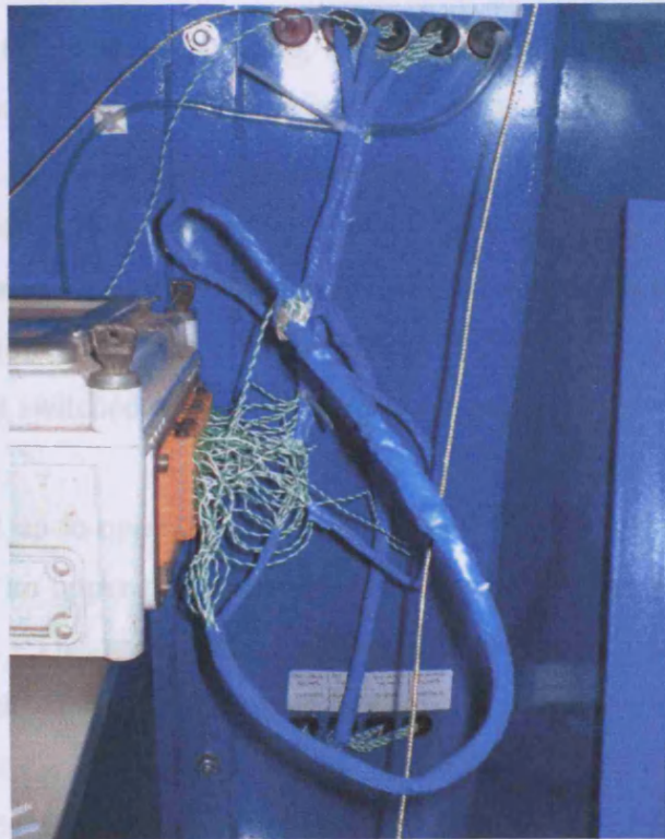
Figure 5.7 Data logger with 49 thermocouples connected via screw terminals.
