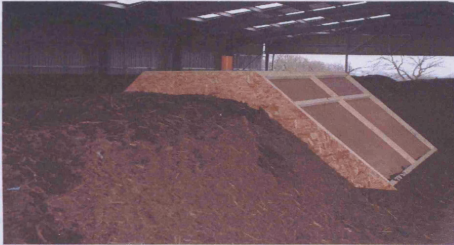
Figure 3.5. Canopy constructed from wood, with 110mm pipe in the top to allow exhaust gases to exit, placed on a green waste windrow.
