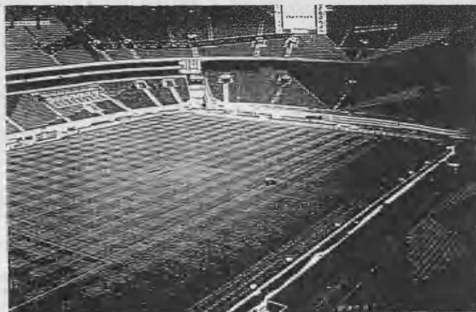
Fig.9.4.5.1.4. The supporting steelwork for the fixed and retractable roof. The hanging steel supports maintenance walkways. The picture reveals the importance of carefully considering a support strategy in considering the contribution that strategy makes in aiding the light flux on the playing surface.
