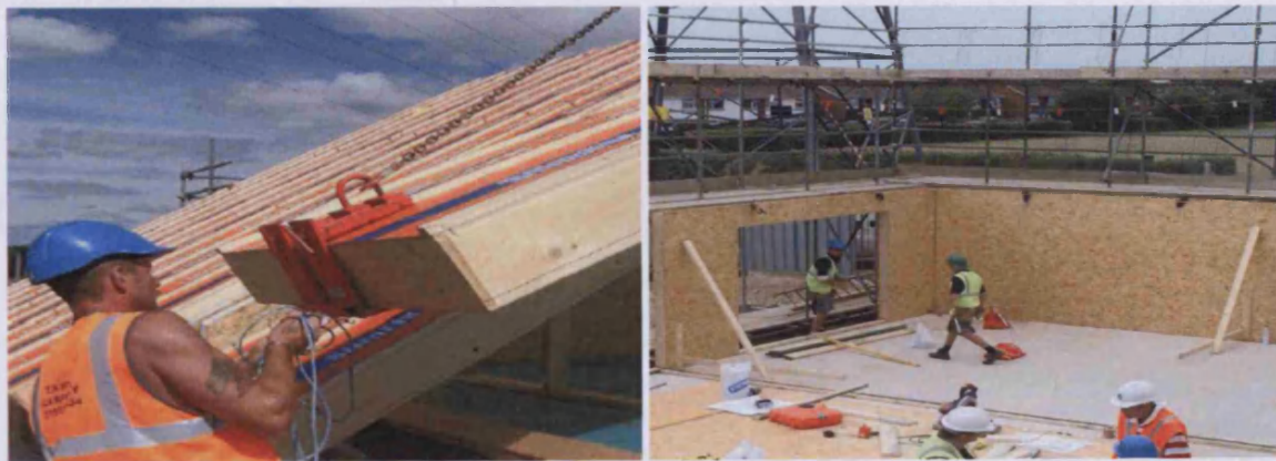
Figure 7-3: Panel system (timber frame) Source: (Hague, 2006)
