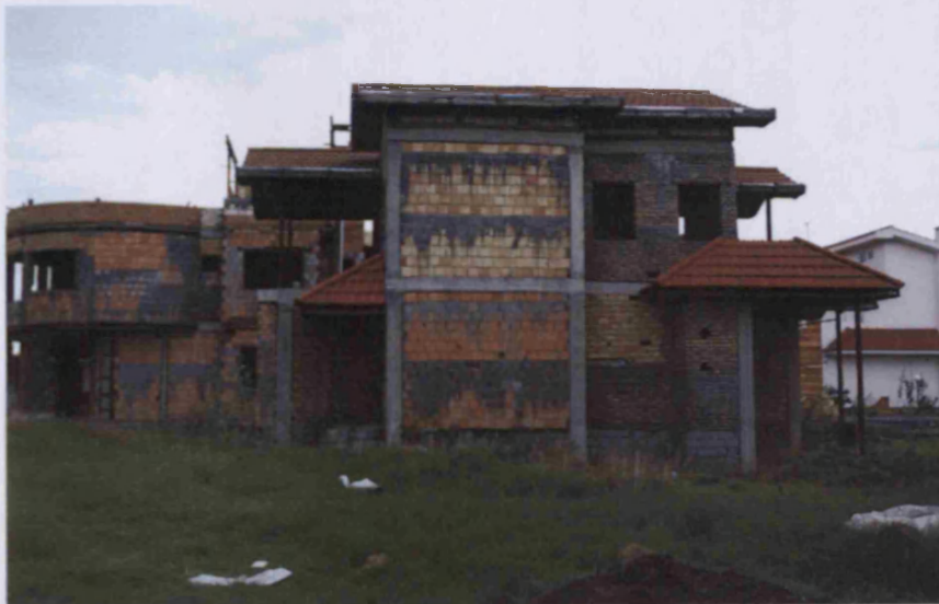
Figure 8-4: Construction methods in north of Iran (RC frame)
