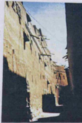
Figure (5-52) Buildings sharing the external wall in three sides kept each other in the shade. Source: Al-Nawaiser (5-11) .
