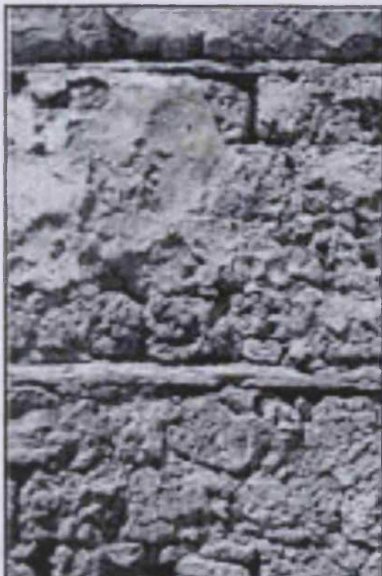
Figure (4-32) The wooden beams construction of the coral wall. Source: King (4-19) .
