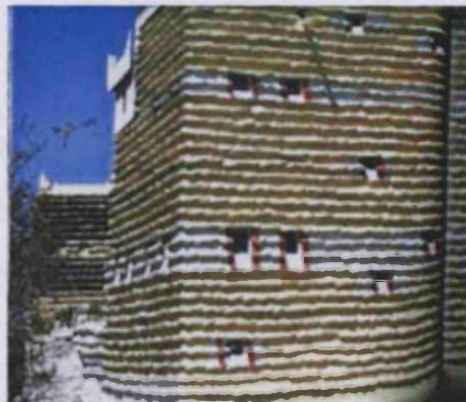
Figure (4-28) Plates of stone overhang outside the buildings as a protection against rain. Source: Al-Hariri and Mauger (4-4, 4-20) .
