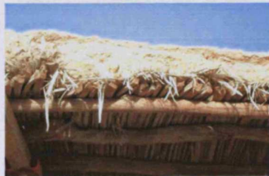
Figure (5-47) The wood and the mud in roof construction of Riyadh houses. Photo by author.
