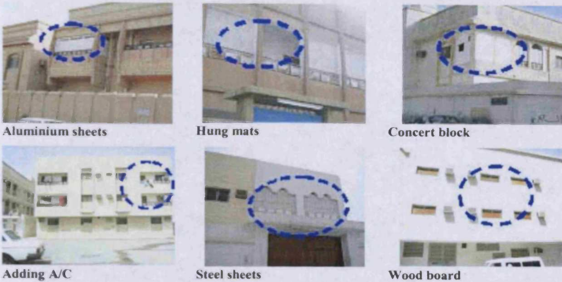
Figure (1-3) Houses modified by inhabitants as a result of poor thermal quality. Photo by author.
