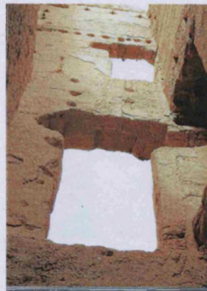
Figure (5-49) The wall thickness about one meter in Dir'yah Area. Source: William Facey (5-7)
