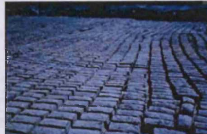
Figure (5-29) Sun dried mud bricks left to be dried in the sun. Photo by author.
