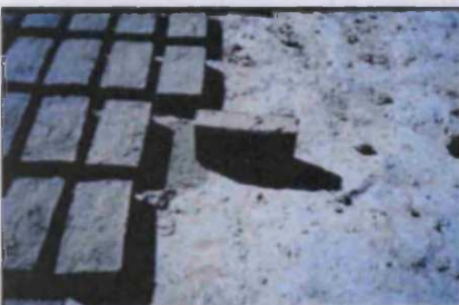
Figure (5-26) The mud brick left to dry in the sun. Photo by author.
