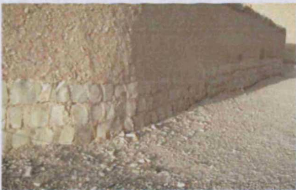
Figure (5-32) Limestone was used in the some building for foundations. Photo by author.
