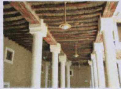
Figure (7-37) The wood trunk carries the roof layer as it constructed in the case studies.
