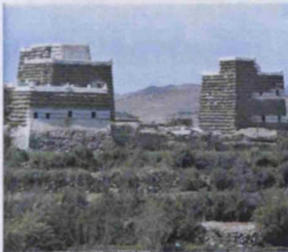
Figure (4-28) Plates of stone overhang outside the buildings as a protection against rain. Source: Al-Hariri and Mauger (4-4, 4-20) .
