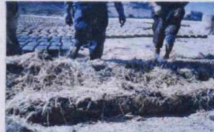
Figure (5-23) Mixed by foot to speed up the process. Photo by author.
