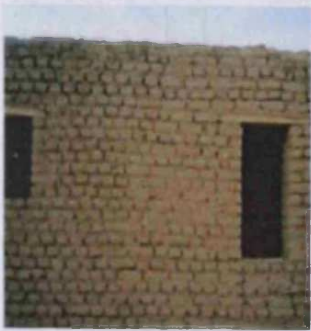
Figure (4-29) Section through the mud wall sun-dried mud brick ( labin ). Source: Mud Construction (4-21) .
