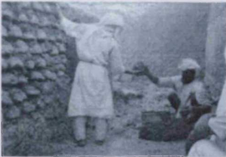
Figure (5-30) Walls constructed by using sun dried mud bricks. Source: AHC. (5-15) .
