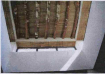
Figure (5-36) The trunk of athel tree used in roof construction. Photo by author.
