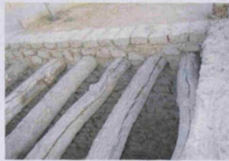
Figure (5-36) The trunk of athel tree used in roof construction. Photo by author.
