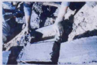
Figure (5-25) Remove wooden mould for other bricks. Photo by author.
