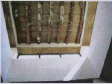
Figure (7-37) The wood trunk carries the roof layer as it constructed in the case studies.
