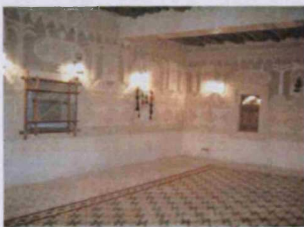
Figure (5-37) Gypsum is the traditional material for plastering. Photo by author.
