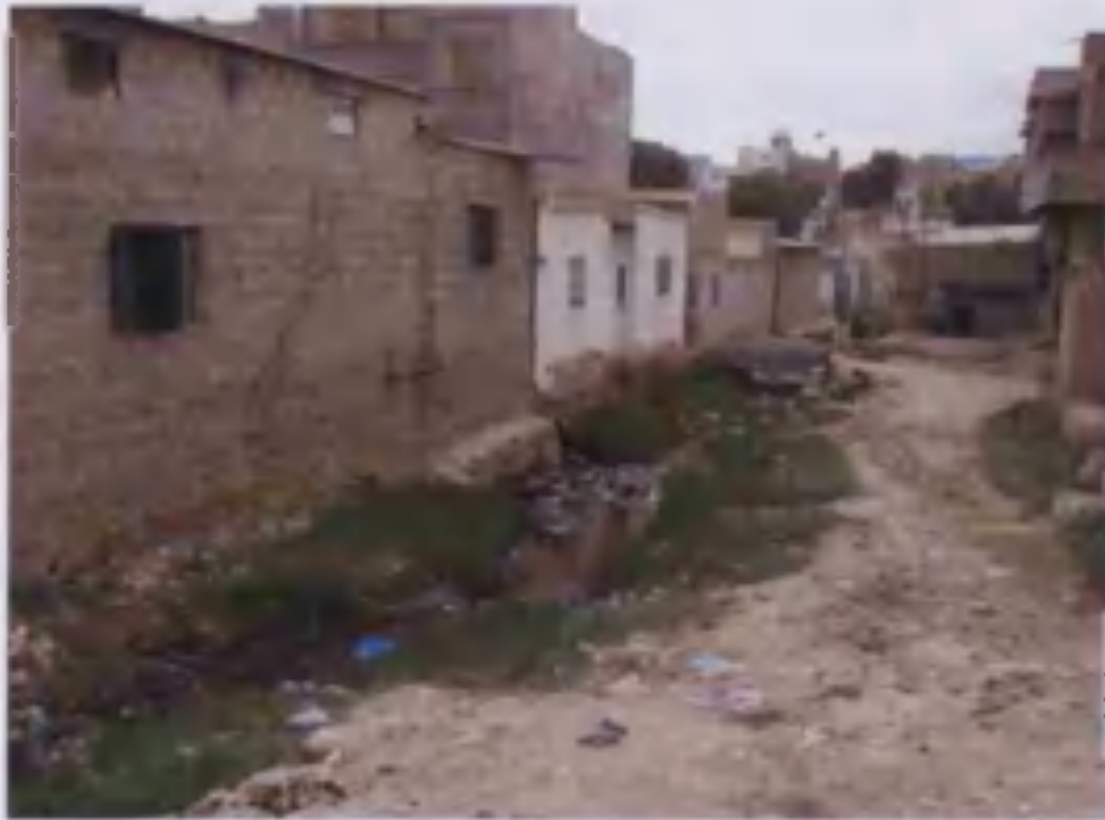
Figure 2.11. Orangi - area without any civic infrastructure
