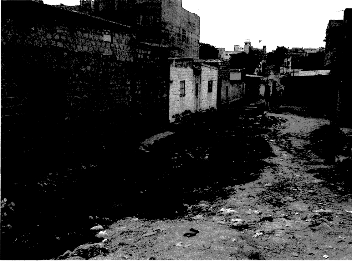
Figure 2.11. Orangi - lane without any civic infrastructure
