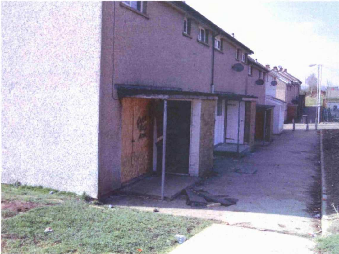
Photograph 2 Derelict houses frequented by young people
