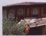
Fig. 5.13: Wada at Pen, originally built:c.1700, Pen, Taluka:Pen, Zilla:Raigad
