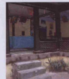
Fig. 5.72: Sahukar Wada, originally built: c.1700, Paithan, Taluka:Paithan, Zilla:Aurangabad
