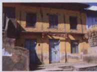
Fig. 5.99: Holkar Wada, originally built: c.1760, Chandwad, Taluka: Chandwad, Zilla: Nasik
