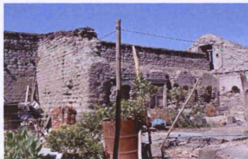
Fig. 4.13: Jadhav Garhi, originally built: c.1700, Bhuins, Zilla: Satara, goshale and kothars in the rear courtyard
