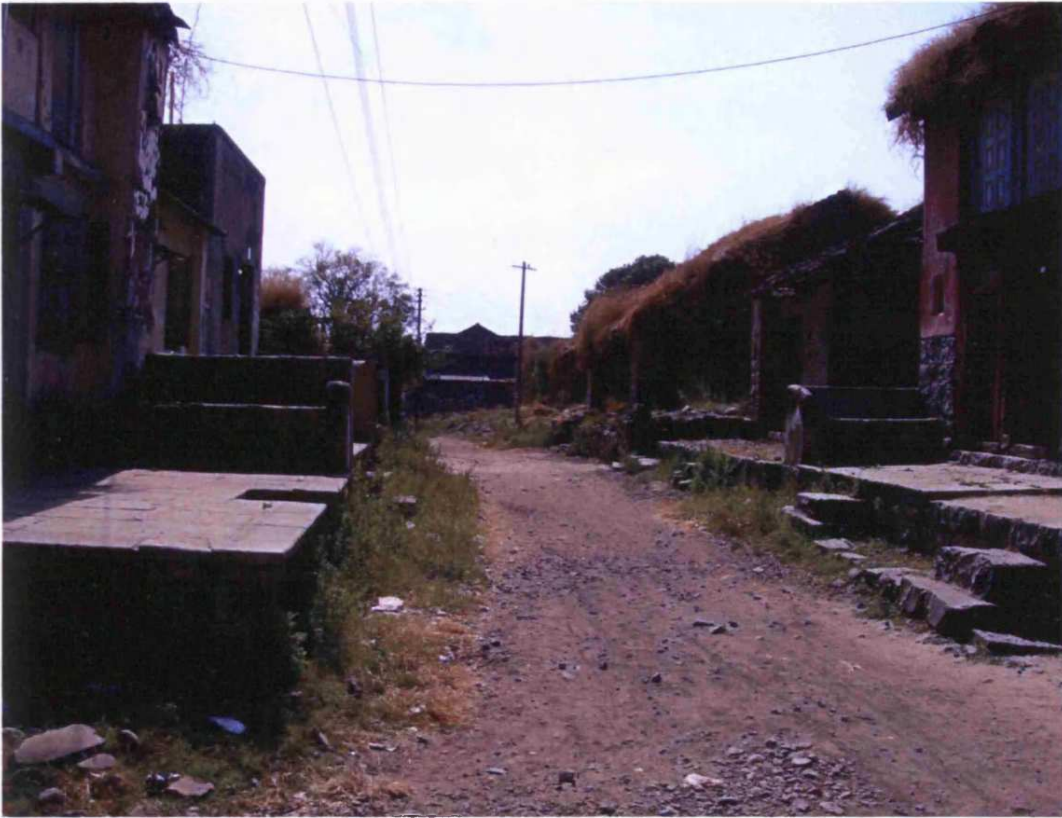
Fig. 8.30: Holkar Wada, Vafgaon, originally built: c.1725, Rajgurunagar, taluka : Khed, Zilla : Pune, Region: Desh, village street
