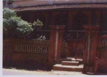
Fig. 5.229: Fallery House, Hari Mandir, originally built: c. 1936, Goa
