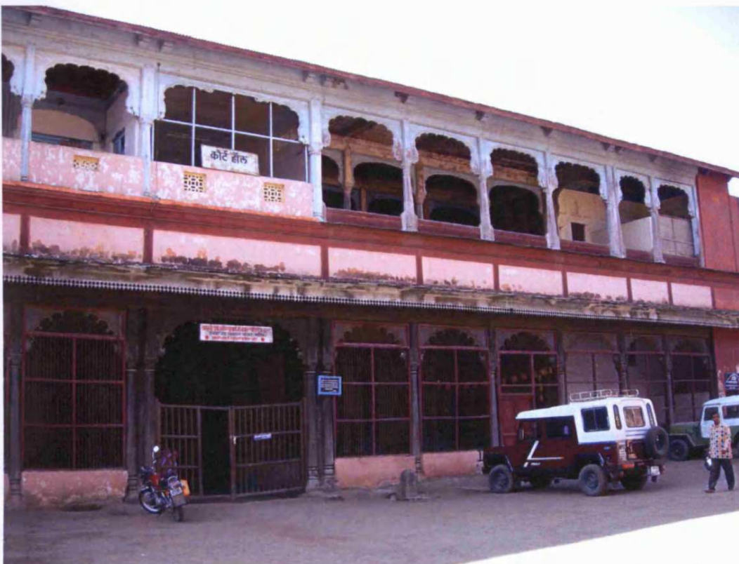
Fig. 8.15: Holkar Wada, originally built: c.1760, Chandwad, Taluka: Chandwad, Zilla: Nasik, Region: Desh, wada within rampart wall
