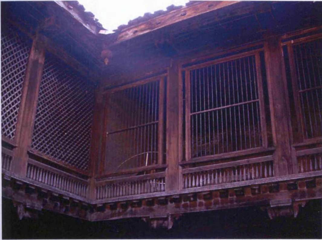
Fig 8.173: Menavli Wada, originally built: c.1768, Menavli, Taluka:Wai, Zilla: Satara, Region:Desh, view of the upper floor from the internal courtyard
