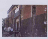
Fig. 5.29: Sridhundiath Maharaj Wada, originally built: c.1650, Paithan, Taluka:Paithan, Zilla:Aurangabad
