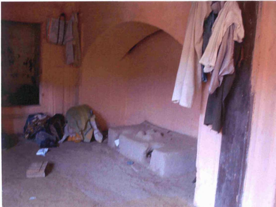
Fig. 8.84: Kadam Wada, originally built c.1700, Taluka:Mulgaon, Zilla: Satara, Region: Desh, cooking area with air vents
