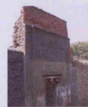
Fig. 5.73: Paithan, originally built: c.1730, Taluka:Paithan, Zilla:Aurangabad
