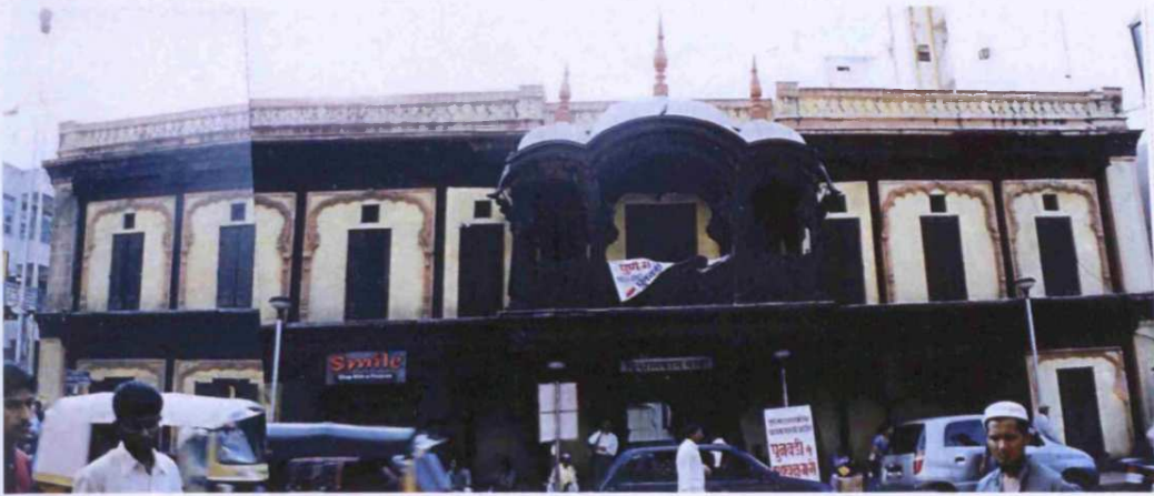
Fig. 3.20: Vishrambagh Wada, originally built: c.1803, Pune, Zilla: Pune, front elevation
