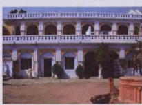
Fig. 5.144: Senior Bhosle Wada, originally built:c. 1840, Nagpur, Taluka:Nagpur, Zilla:Nagpur, Region:Vidharbha
