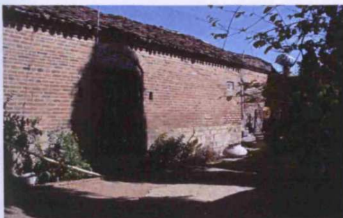
Fig. 4.14: Jadhav Garhi, originally built: c.1700, Bhuins, Zilla: Satara, well in the courtyard
