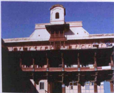
Fig. 2.6: Holkar Wada, originally built: c.1760, Chandwad, Taluka: Chandwad, Zilla: Nasik, Region: Desh, elevation of first internal courtyard
