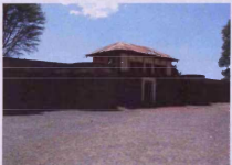
Fig. 5.143: Kadam Wada, originally built: c.1700,Sap Taluka:Mulgaon, Zilla:Satara, Region:Desh
