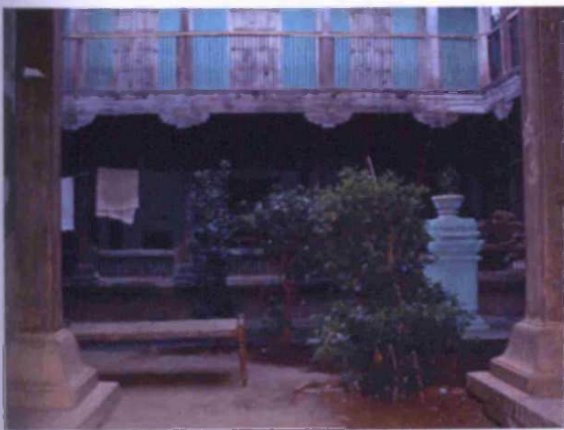
Fig. 6.29: Mohite Wada, originally built: c.1700, Rajewadi, Taluka: Rajewadi, Zilla: Satara, Region: Desh, , view of tulsi vrindavan in courtyard.
