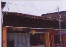
Fig. 5.219: Wada at Pimpalner, originally built: c.1725, Taluka:Sakri, Zilla:Dhule
