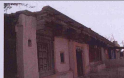
Fig. 5.172: Phadnis Wada, originally built: c.1700, Srigonda, Taluka:Srigonda, Zilla:A Ahmednagar, Region:Desh
