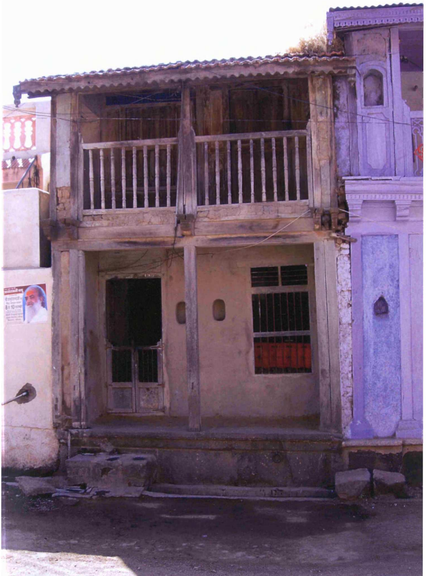
Fig. 8.13: Holkar Wada, originally built: c.1760, Chandwad, Taluka: Chandwad, Zilla: Nasik, Region: Desh, street façades around fort
