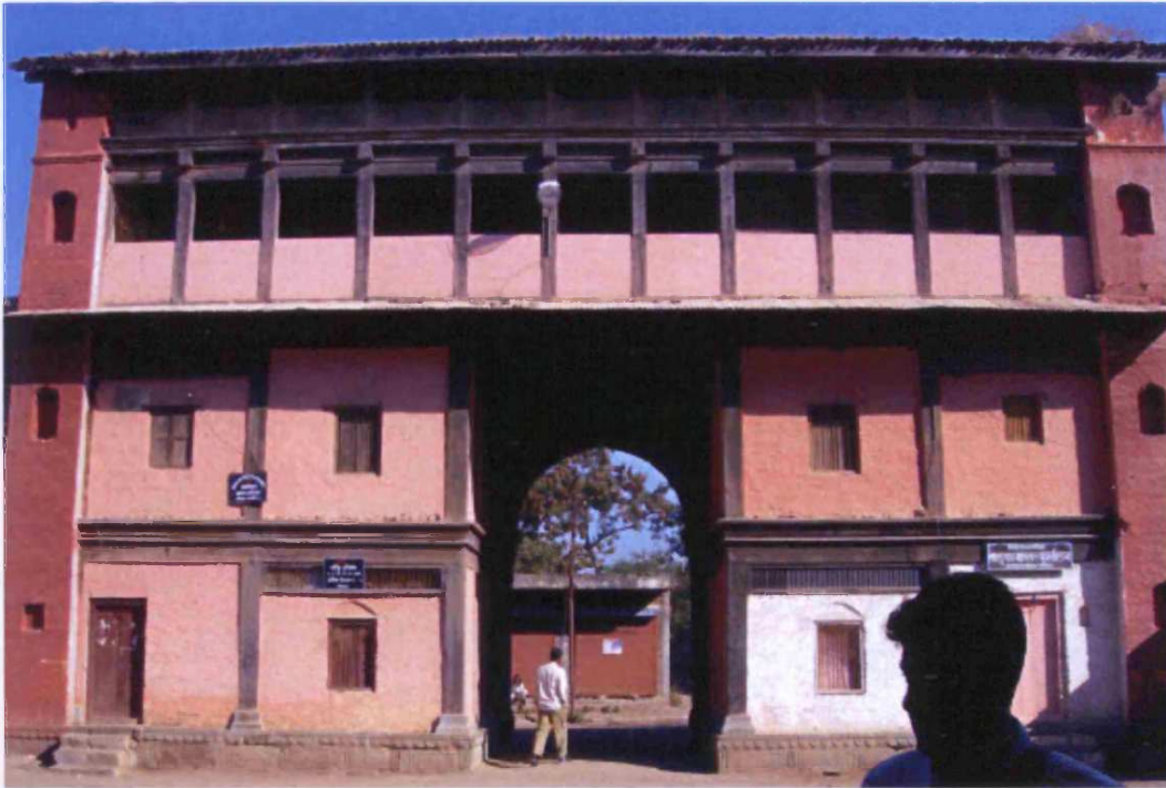
Fig. 8.14: Holkar Wada, originally built: c.1760, Chandwad, Taluka: Chandwad, Zilla: Nasik, Region: Desh, elevation first internal courtyard
