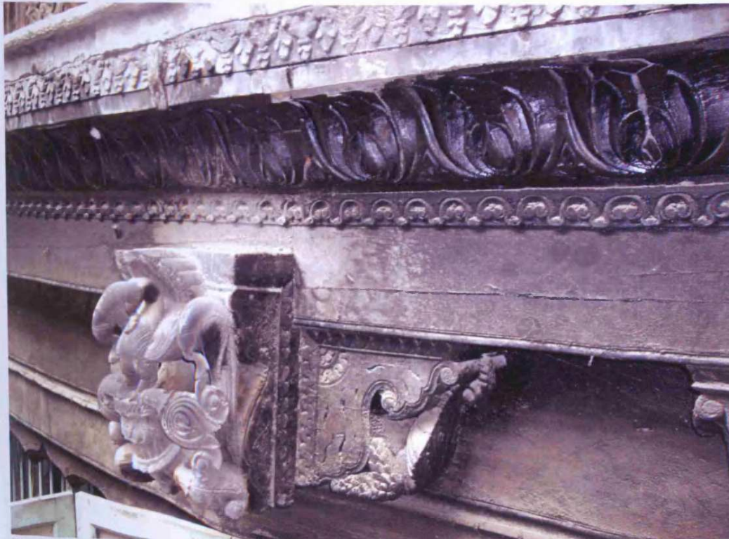
Fig. 8.124: Vishrambagh Wada, Pune, originally built: c.1803, Taluka: Pune, Zilla: Pune, Region: Desh, slap, fascia and beam head detail
