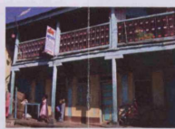
Fig. 5.34: Wada at Pimpalner, originally built: c.1725, Pimpalner Taluka:Sakri, Zilla:Dhule
