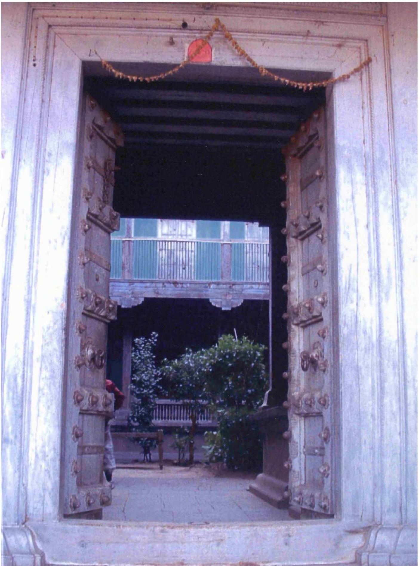
Fig. 8.128: Senapati Mohite Wada, originally built: c.1700, Rajewadi, Taluka: Khandala, Zilla: Satara, Region: Desh, view into the internal courtyard
