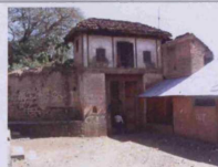
Fig. 5.154: Wada at Menavli, originally built: c.1768, Menavli, Taluka:Wai, Zilla:Satara, Region:Desh
