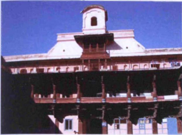
Fig. 6.23: Holkar Wada, originally built:c.1760, Chandwad, Taluka: Chandwad, Zilla:Nasik, Region: Desh Desh, elevation, first internal courtyard
