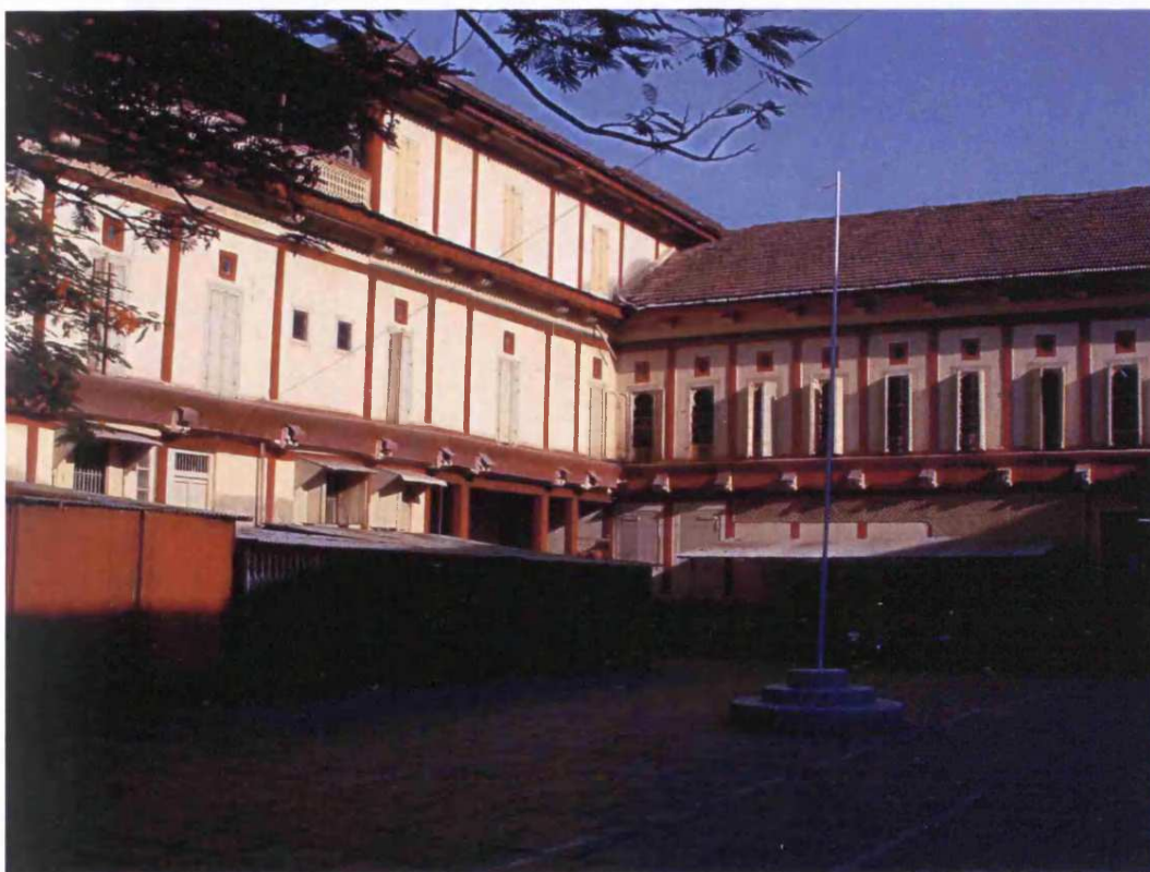
Fig. 8.111: Rajwada, originally built: c.1700, Taluka: Satara, Zilla: Satara, Region: Desh, main courtyard
