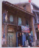
Fig. 5.221: Wada at Pimpalner, originally built: c.1725, Taluka:Sakri, Zilla:Dhule
