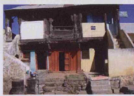
Fig. 5.90: Pingte Wada, originally built: c.1760, Chandwad, Taluka:Chandwad, Zilla:Nasik
