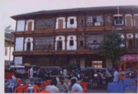
Fig. 5.74: Rajwada, originally built: c.1700, Satara, Taluka:Satara, Zilla:Satara
