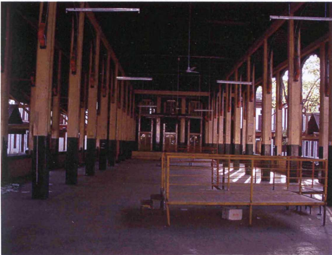
Fig. 8.116: Rajwada, originally built: c.1700, Taluka: Satara, Zilla: Satara, Region: Desh, pillared hall, sofa in courtyard
