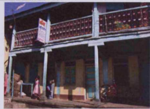
Fig. 5.217: Wada at Pimpalner, originally built: c.1725, Taluka:Sakri, Zilla:Dhule
