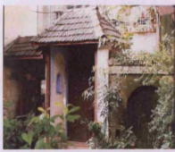
Fig. 5.22: Sathe Wada, originally built: c.1874, Kalyan, Taluka:Kalyan, Zilla:Thane
