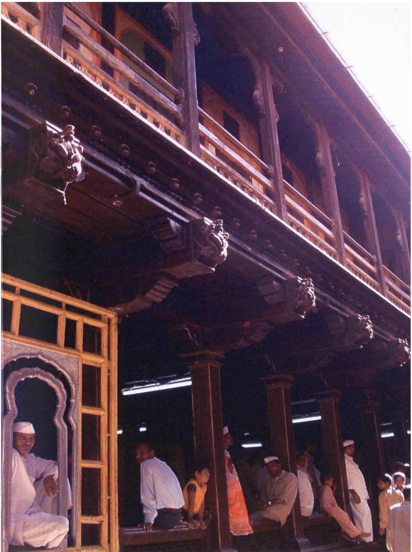
Fig. 8.101: Bhor Rajwada, originally built: c.1750, Bhor, Taluka: Pune, Zilla: Pune, detail of cantilevered projection, supported by wooden brackets
