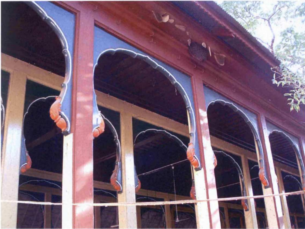
Fig. 8.115: Rajwada, originally built: c.1700, Taluka: Satara, Zilla: Satara, Region: Desh, detail of wooden Peshwai arches in the sofa
