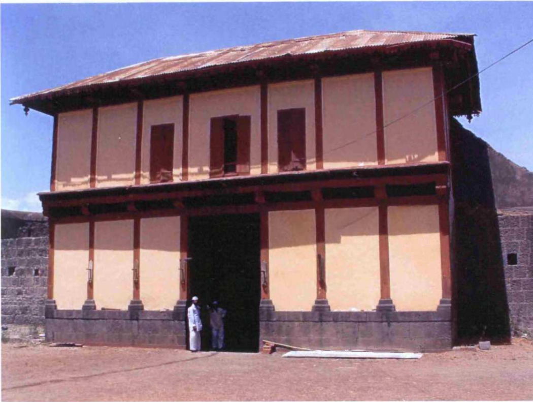
Fig. 8.71: Kadam Wada, originally built c.1700, Taluka:Mulgaon, Zilla: Satara, Region: Desh, view from the internal courtyard towards the main entrance
