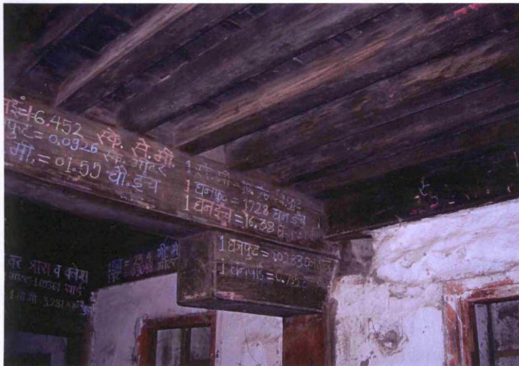
Fig. 8.22: Holkar Wada, originally built: c.1760, Chandwad, Taluka: Chandwad, Zilla: Nasik, Region: Desh, wooden ceiling showing main beams and cross beams
