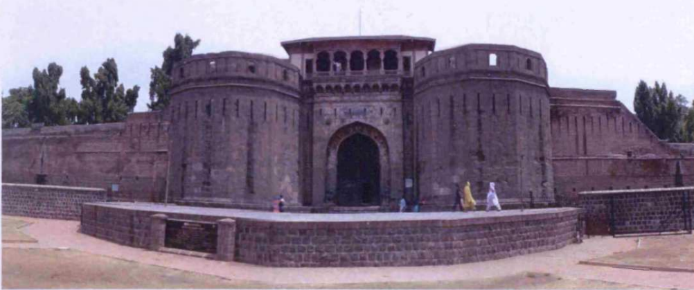
Fig. 3.17: Shaniwar Wada, originally built: c.1736, Pune, Zilla: Pune, main entrance with bastions and ramparts
