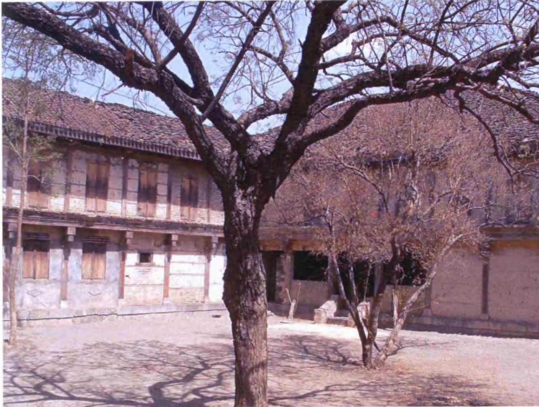
Fig. 8.62: Purandhare Wada, Modwa, originally built: c.1700, Taluka: Baramati, Zilla: Pune, Region: Desh, built form overlooking the main courtyard
