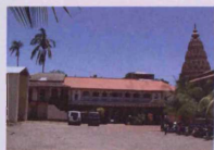
Fig. 5.75: Rajwada, originally built: c.1829, Aundh, Taluka:Koregaon, Zilla:Satara
