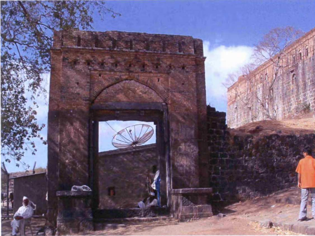
Fig. 8.51: Jadhav Rao Garhi, originally built: c.1600, Taluka: Purandhar, Zilla: Pune, Region: Desh, entrance gateway into the goshala
