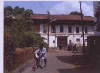
Fig. 5.149: Datar Wada, originally built: c.1725, Pen, Taluka:Pen, Zilla:Raigad, Region:Konkan
