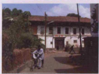
Fig. 5.31: Datar Wada, originally built: c.1725, Pen, Taluka:Pen, Zilla:Raigad
