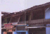
Fig. 5.35: Wada at Pimpalner, originally built: c.1725, Pimpalner, Taluka:Sakri, Zilla:Dhule
