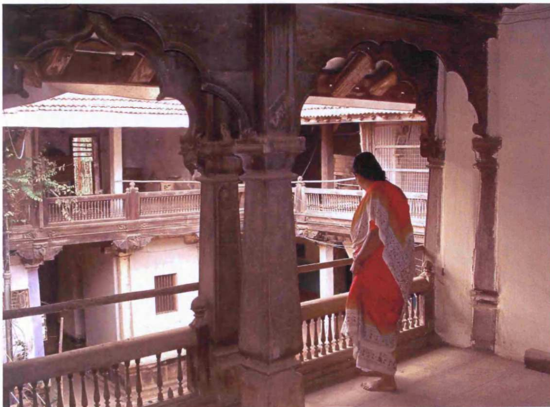
Fig. 8.142: Datar Wada, originally built: c.1725, Taluka: Pen, Zilla: Raigad, Region: Konkan, Peshwai arches overlooking main courtyard
