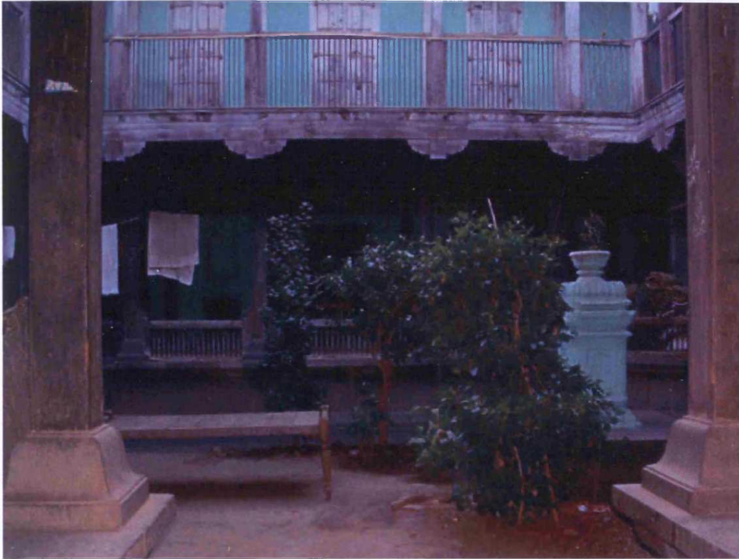
Fig. 8.130: Senapati Mohite Wada, originally built: c.1700, Rajewadi, Taluka: Khandala, Zilla: Satara, Region: Desh, view of tulsī vrindavan in courtyard
