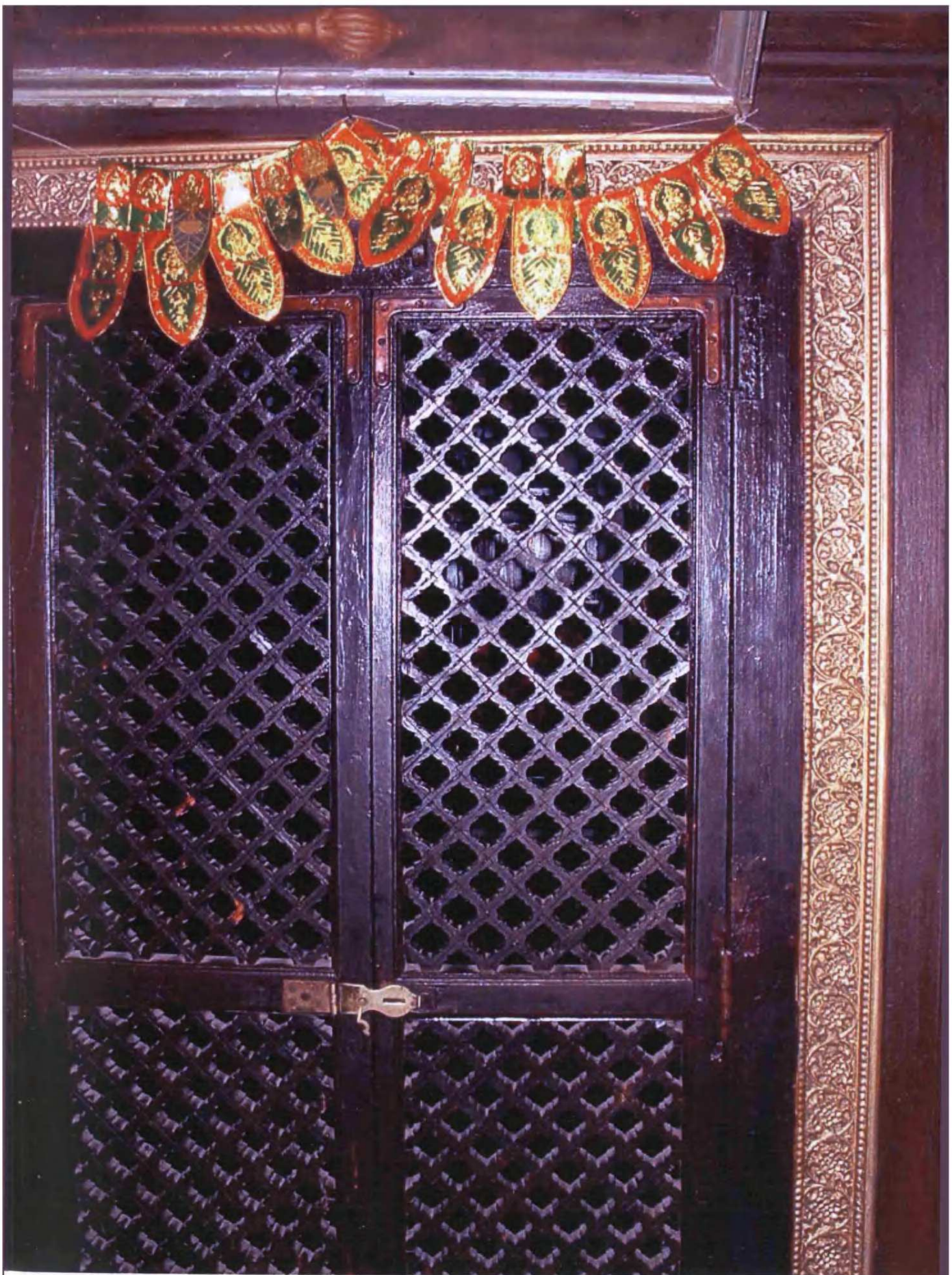
Fig. 8.104: Bhor Rajwada, originally built: c.1750, Bhor, Taluka: Pune, Zilla: Pune, wooden jali door and deoghar
