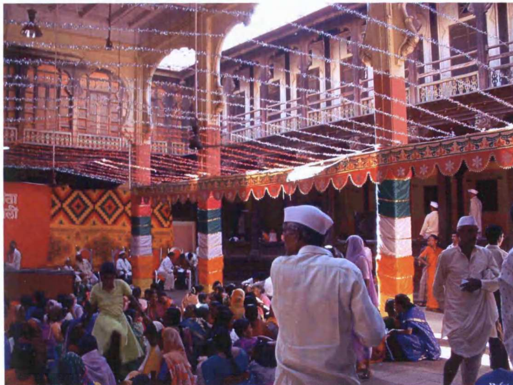
Fig. 8.98: Bhor Rajwada, originally built: c.1750, Bhor, Taluka: Pune, Zilla: Pune, view from internal court
