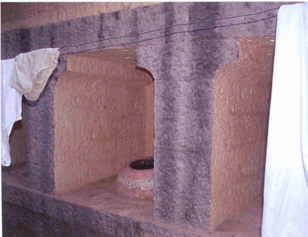
Fig 8.94: Mahadji Shinde Wada , originally built: c.1700, Taluka: Srigonda, Zilla: Ahmednagar, Region: Desh, earthenware pots for water storage
