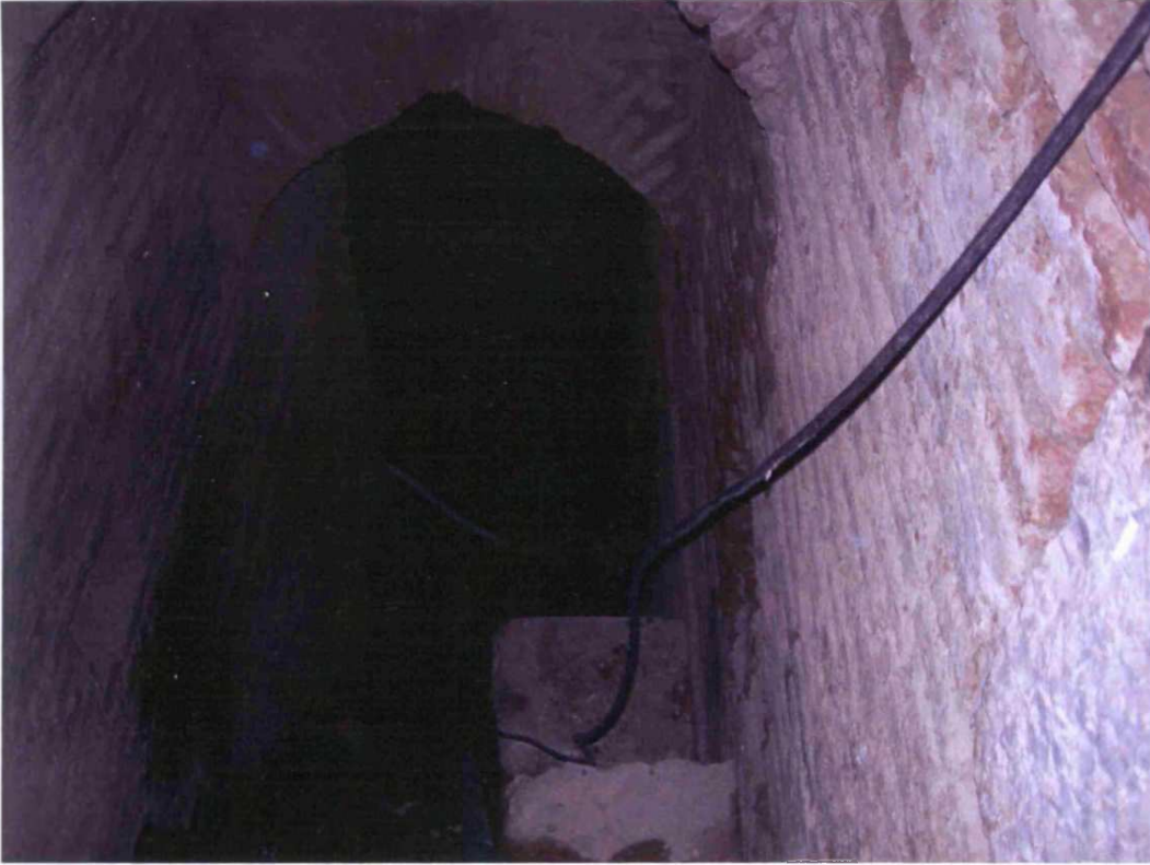
Fig. 8.46: Holkar Wada, Vafgaon, originally built: c.1725, Rajgurunagar, taluka: Khed, Zilla: Pune, Region: Desh, stepwell
