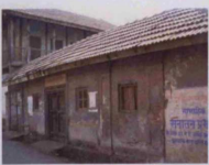
Fig. 5.11: Patwardhan Wada, originally built: c.1750, Panvel, Taluka:Panvel, Zilla:Raigad
