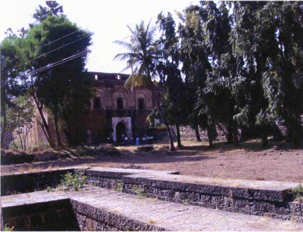
Fig. 8.35: Holkar Wada, Vafgaon, originally built: c.1725, Rajgurunagar, taluka: Khed, Zilla: Pune, Region: Desh, courtyard
