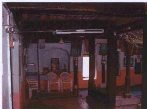
Fig. 4.9: Patil Wada, originally built: c.1700, Paithan, Taluka: Paithan, Dist: Aurangabad, sopa abutting internal court
