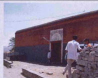
Fig. 5.181: Mahurkar Wada, originally built: c.1870, Mahur, Taluka:Purandhar, Zilla:Pune, Region:Desh
