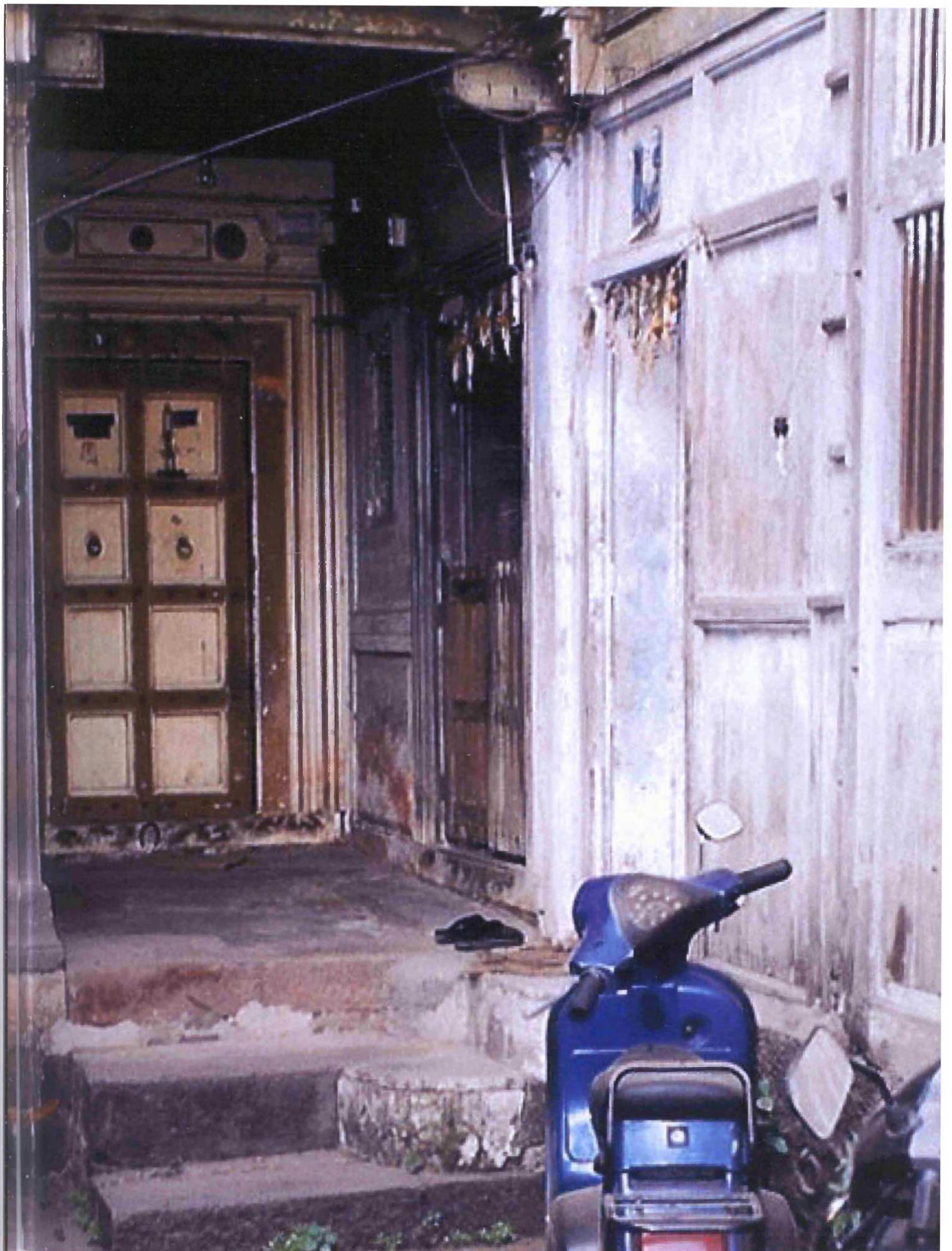
Fig. 8.150: Joshi Wada, Kalyan, originally built: c.1850, Old Kalyan, Taluka: Kalyan, Zilla:Thane, Region: Konkan, main courtyard
