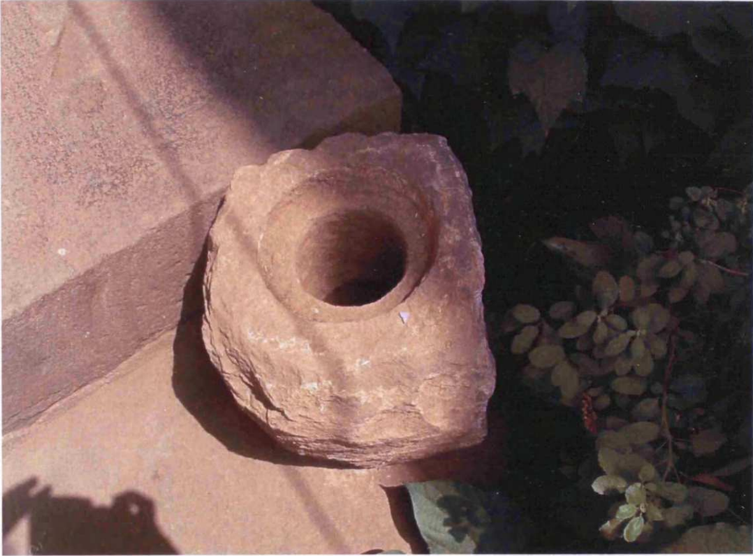
Fig. 8.145: Datar Wada, originally built: c.1725, Taluka: Pen, Zilla: Raigad, Region: Konkan, part of stone drainage pipe with interlocking detail
