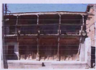
Fig. 5.98: Brahmin Wada, originally built: c.1760, Chandwad, Taluka:Chandwad, Zilla:Nasik
