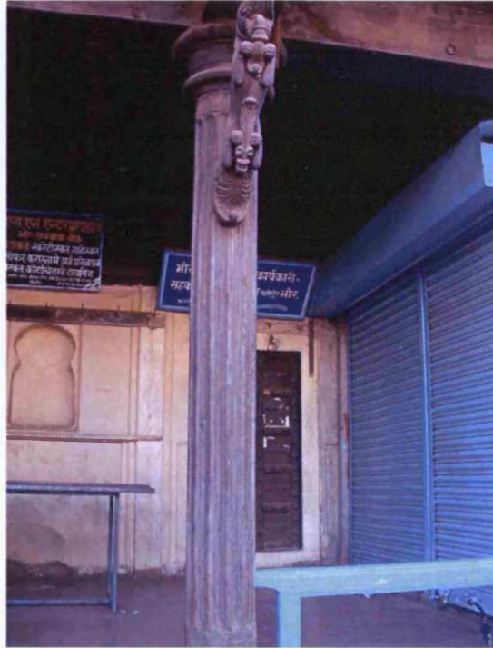
Fig. 8.108: Bhor Rajwada, originally built: c.1750, Bhor, Taluka: Pune, Zilla: Pune, wooden with bracket in devadi
