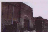
Fig. 5.32: Purandhare Wada, originally built: c.1700, Modva, Taluka:Baramati, Zilla:Pune
