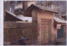
Fig. 5.159: Shedge Wada, originally built c.1800, Panvel, Taluka:Panvel, Zilla:Raigad, Region:Konkan
