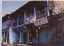
Fig. 5.220: Wada at Pimpalner, originally built: c.1725, Taluka:Sakri, Zilla:Dhule
