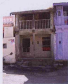
Fig. 5.103: Holkar Wada, originally built: c.1760, Chandwad, Taluka:Chandwad, Zilla:Nasik
