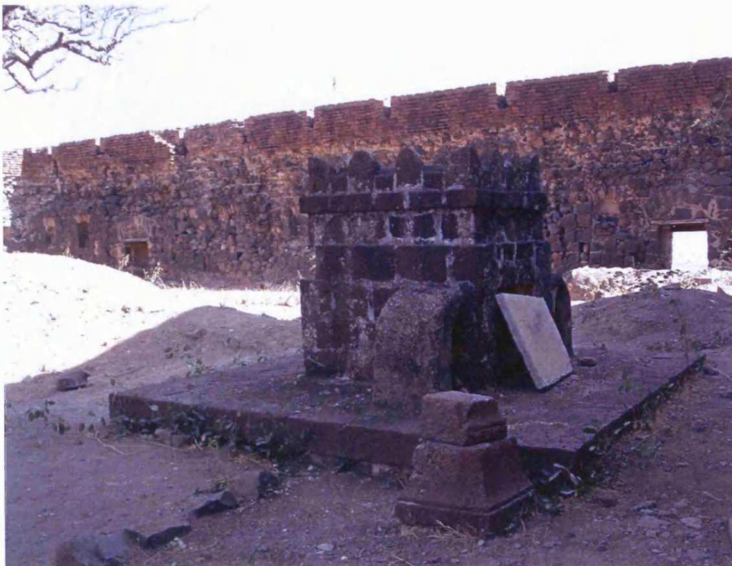
Fig. 8.56: Jadhav Rao Garhi , originally built: c.1600, Taluka: Purandhar, Zilla: Pune, Region: Desh, internal courtyard with tulsi vrindavan
