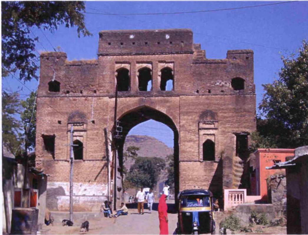
Fig. 8.11: Holkar Wada, originally built: c.1760, Chandwad, Taluka: Chandwad, Zilla: Nasik, Region: Desh, gateway of town wall
