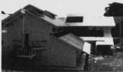
Figure 4: The chimneys of the Queens building at DeMontfort University provide the exhaust for the naturally ventilated lecture theatres and other teaching spaces
