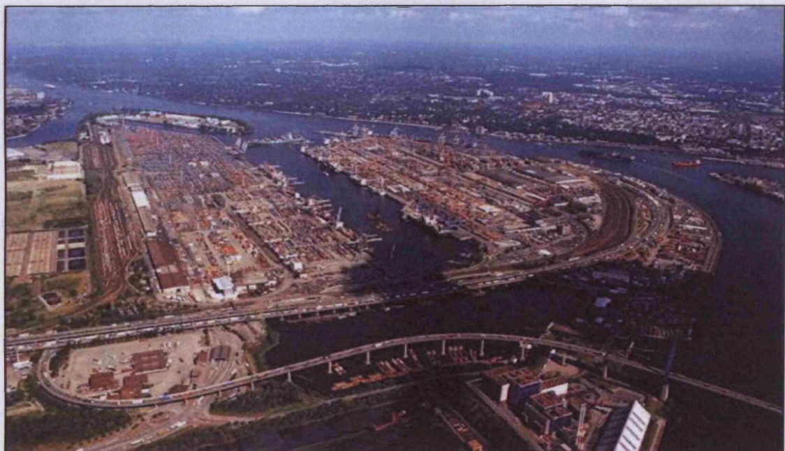
Figure 71: Container Terminals Waltershof – Port of Hamburg
