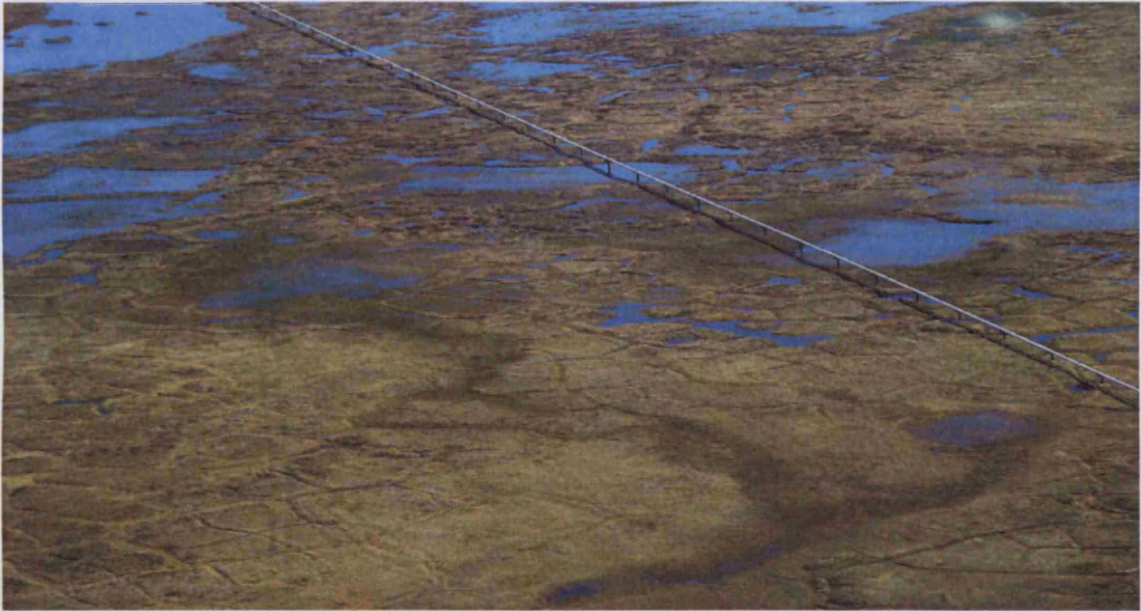
Figure 44: Oil pipeline on central North Slope coastal plain, Alaska
