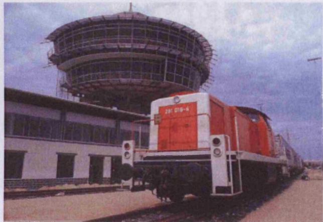
Figure 72: PRIOS Control tower
