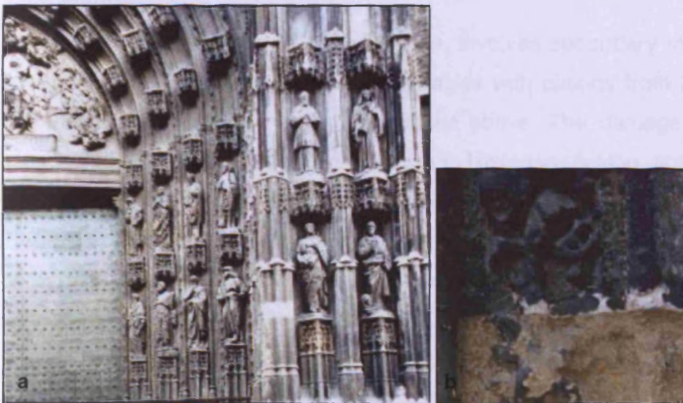
Figure 6 Black crust on Seville cathedral a. Thick black crust, with detail (b), on Seville cathedral, Spain with hydrocarbon-degrading microorganisms (Saiz-Jimenez, 1995).
