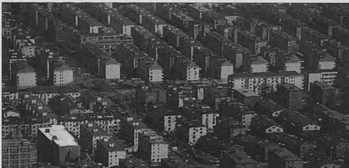
Figure 4.16 Work-unit compounds sprawling across vast urban areas, Shanghai: they became the principal urban space unit during the Maoist period (Denison and Ren 2005).
