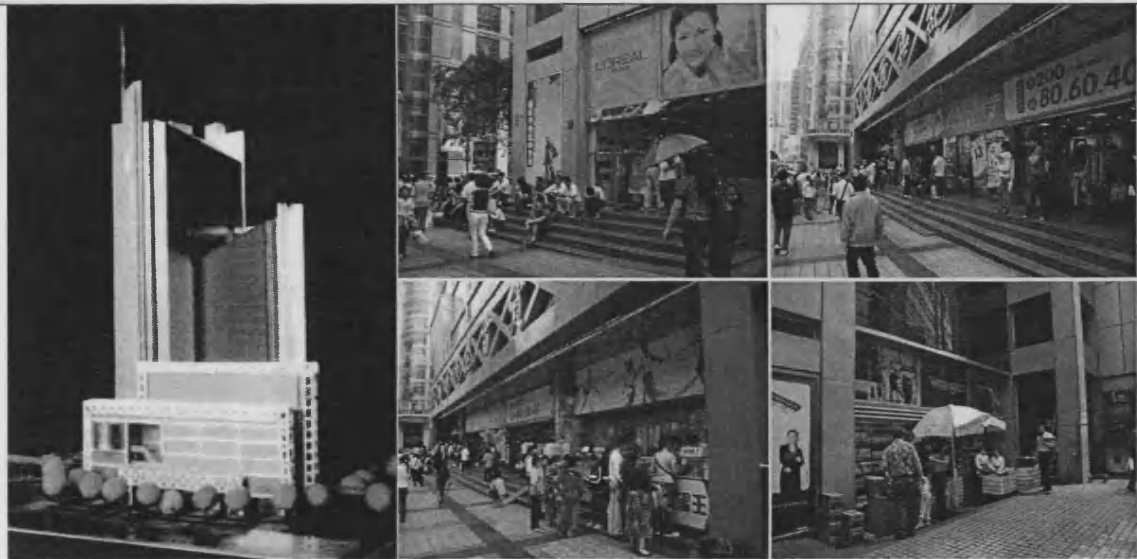
Figure 6.11 New Century Mansion (Source: Dai Zhizhong; photo taken by the author).
